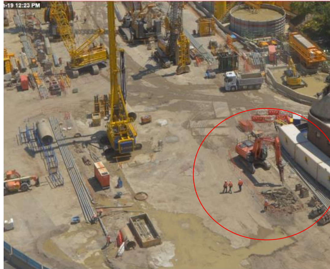
Northern section of works
