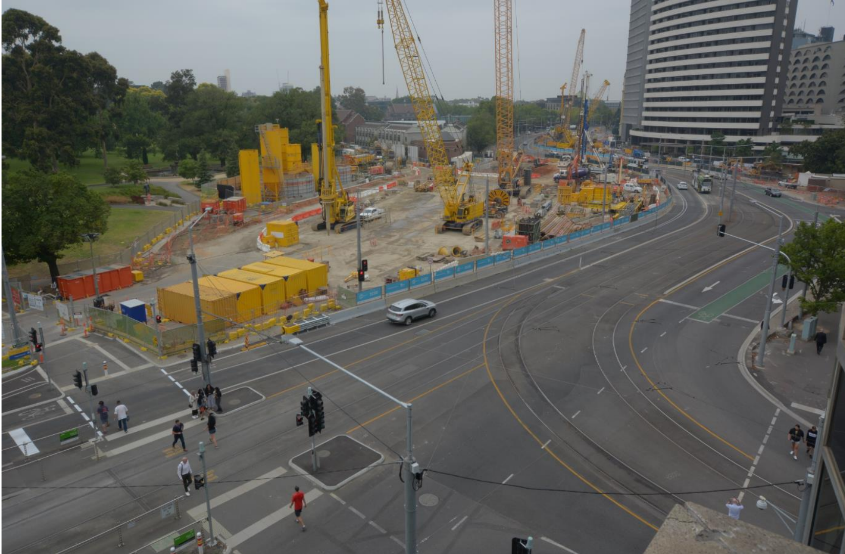
Timelapse image of north section station box works
