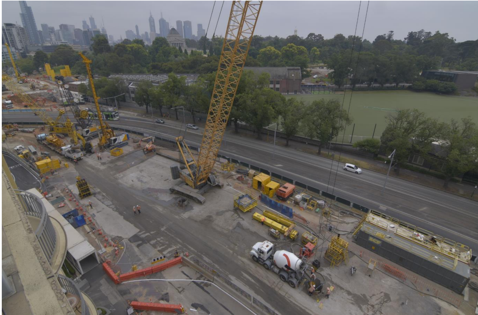
Timelapse image of southern station box works
