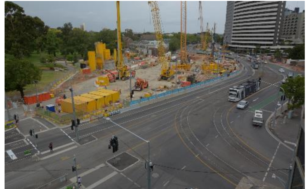
Northern section of works
