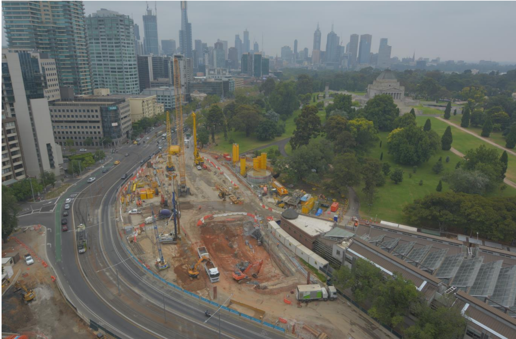
Timelapse image of northern station box works
