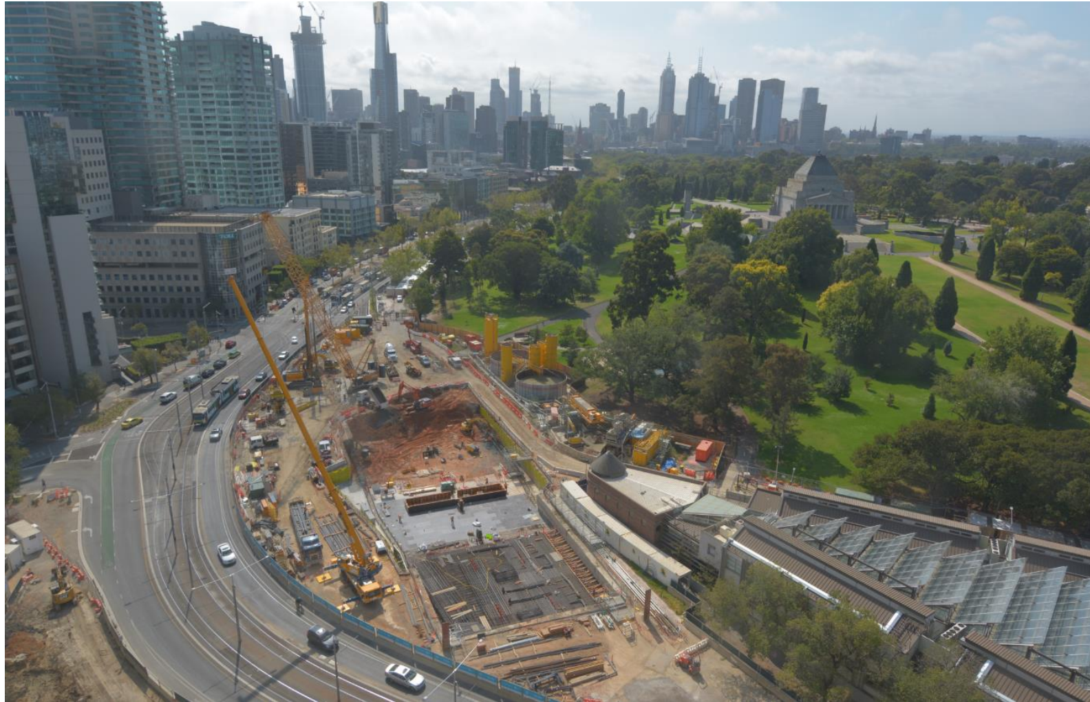
Timelapse image of northern station box works
