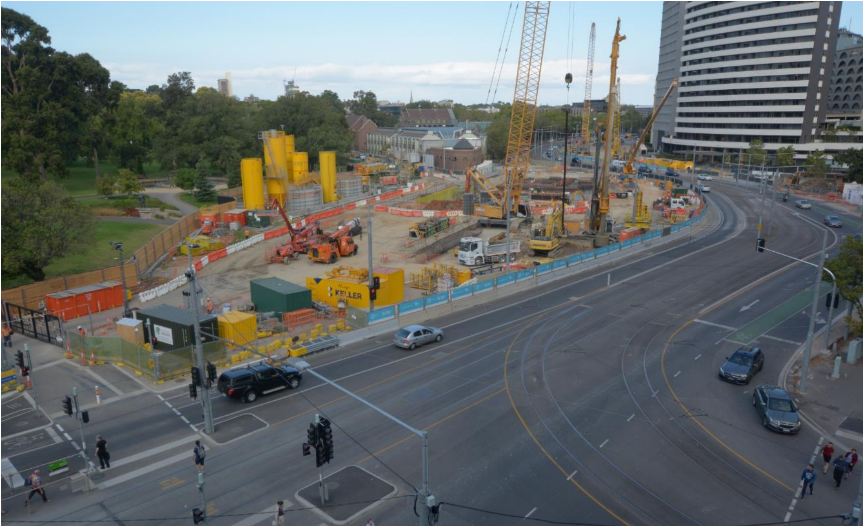
Timelapse image of northern station box works
