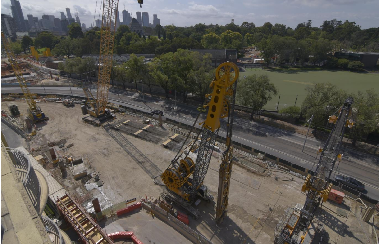
Timelapse image of southern station box works
