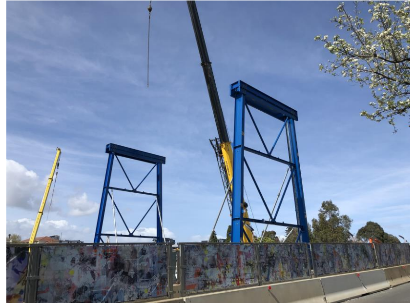
Gantry crane construction Osborne Street
