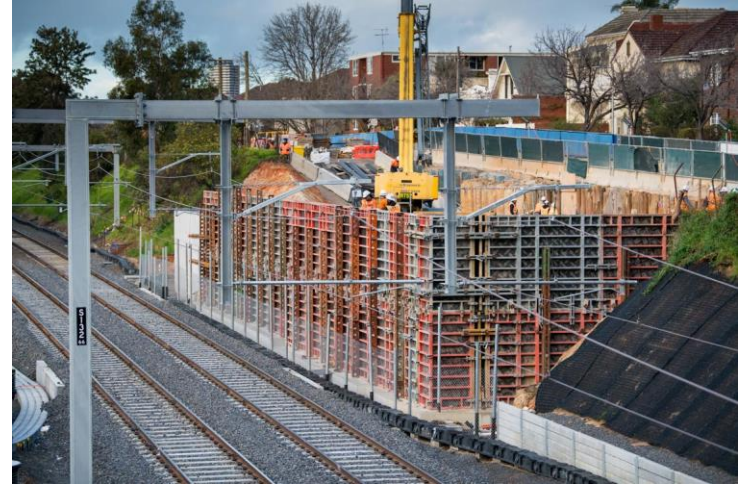
Formwork at Osborne Street site
