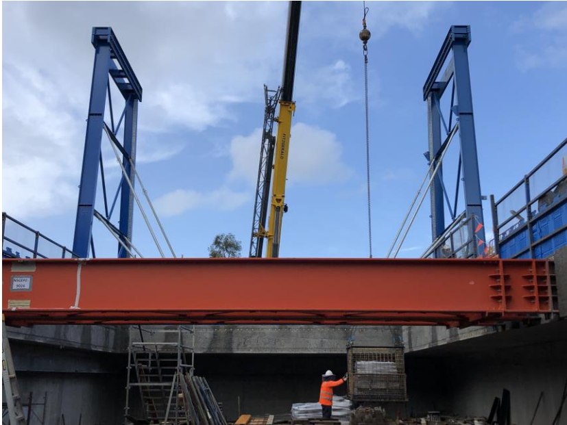
Gantry crane construction Osborne Street
