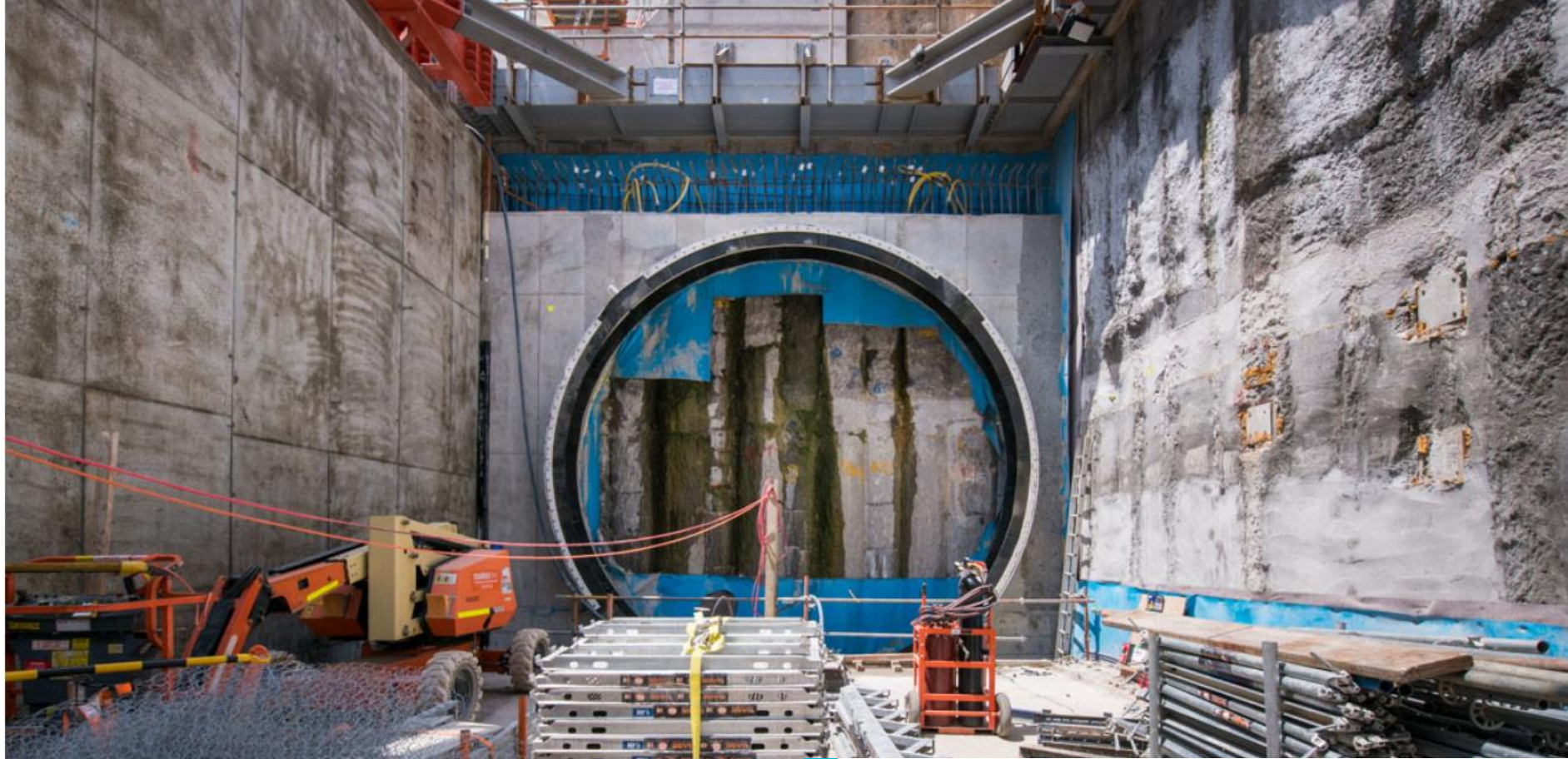
DIVIDING WALL AND RECEPTION SEAL
