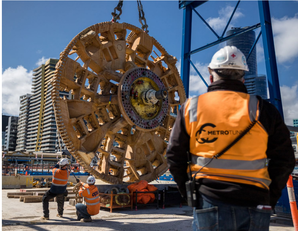
TBM Millie's cutterhead lift
