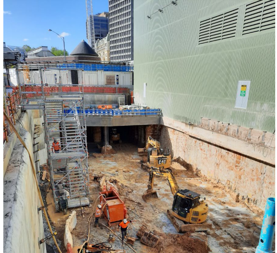
The excavation and completed section of roof slab
