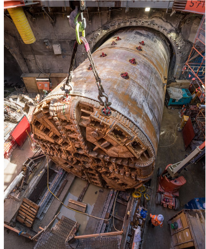
TBM Millie prior to the cutterhead lift
