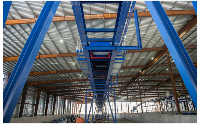
Above: The fit out of the spoil handling facility at the Tunnelling Hub (221 Whitehall Street) is almost complete. The blue steel is the spoil conveyor being constructed.
