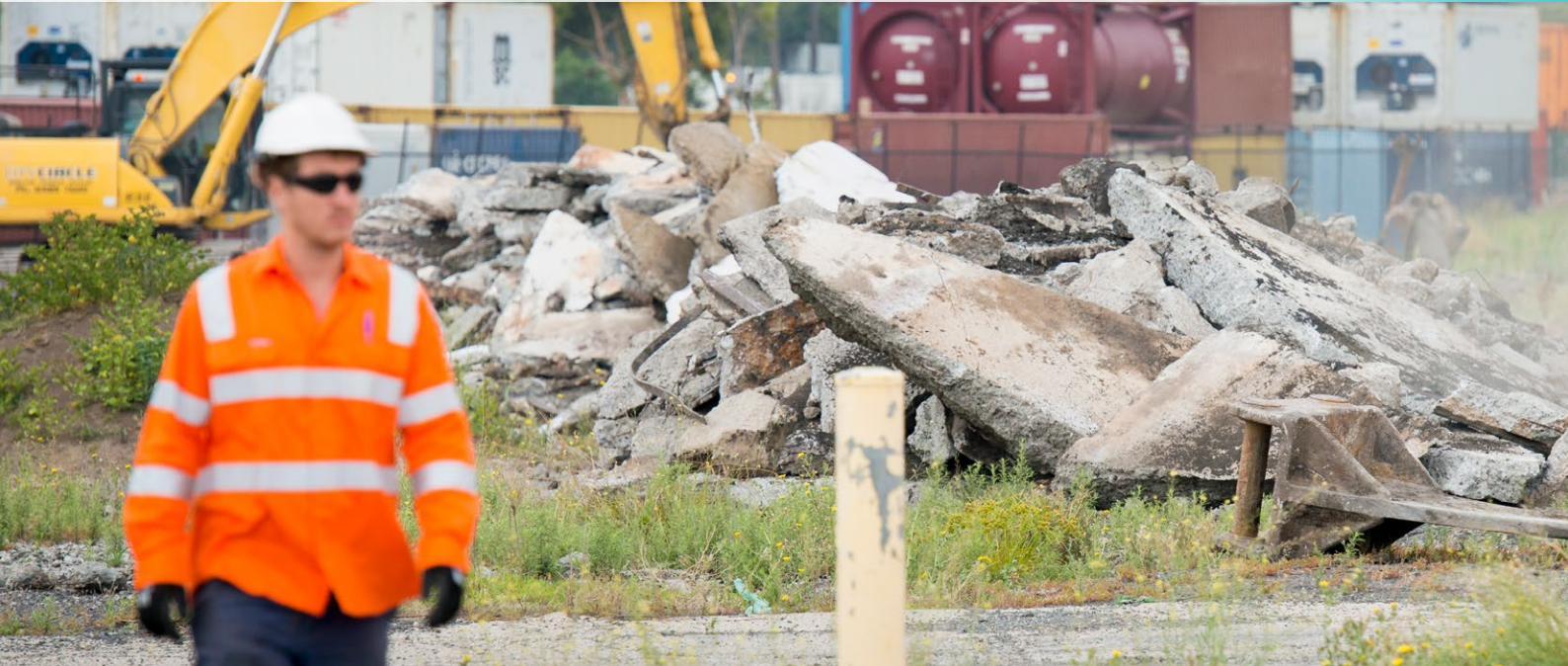
Works at the Northern Portal, Footscray.
