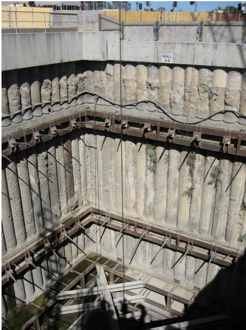
Figure 3-2 Anchored and braced bored pile retaining walls (Airport Link, Brisbane, 2011)
