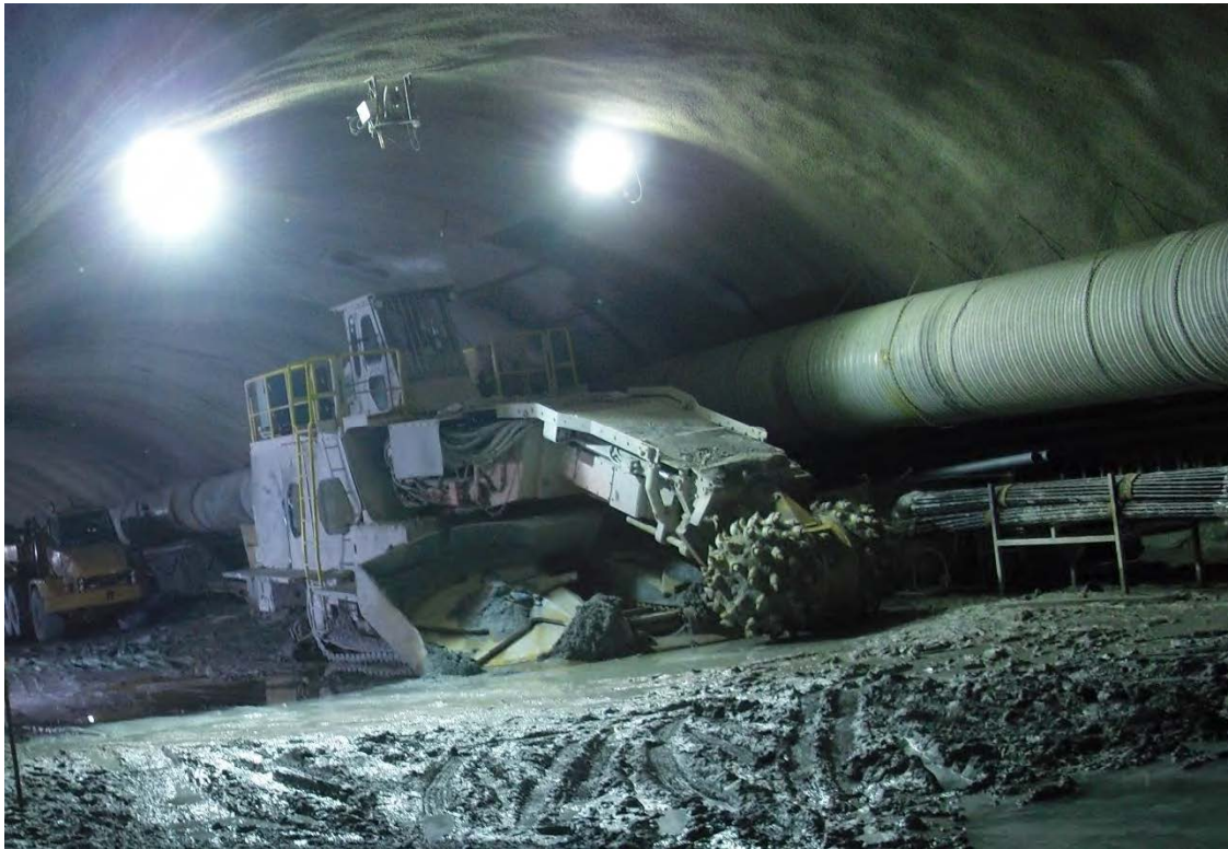
Figure 3-5 SEM tunnelling with roadheader (Airport Link, Brisbane, 2010)
