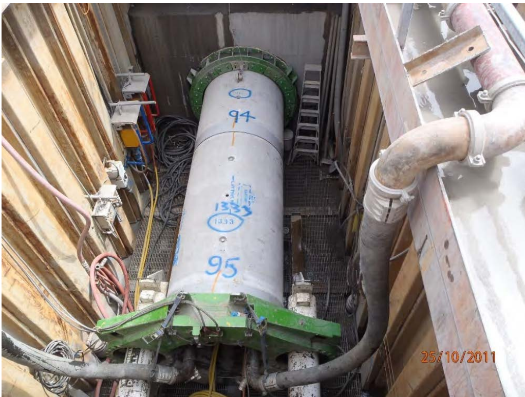
Figure 3-6 Pipe-jacking for a new sewer (Christchurch, 2011)
