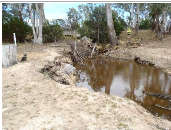
Figure 21: Donald Creek, upstream of the existing highway culvert.
