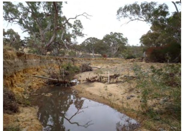
Figure 4: Concongella Creek approximately 150 m downstream of existing Highway culverts
