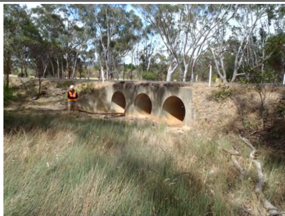
Figure 15: Upstream view of culverts
