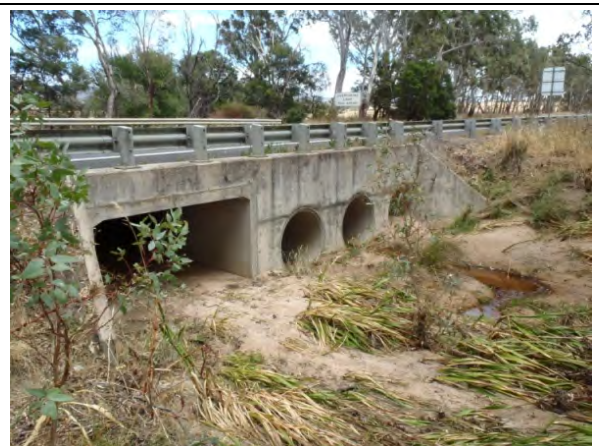
Figure 22: Donald Creek, looking upstream at the existing highway culvert.
