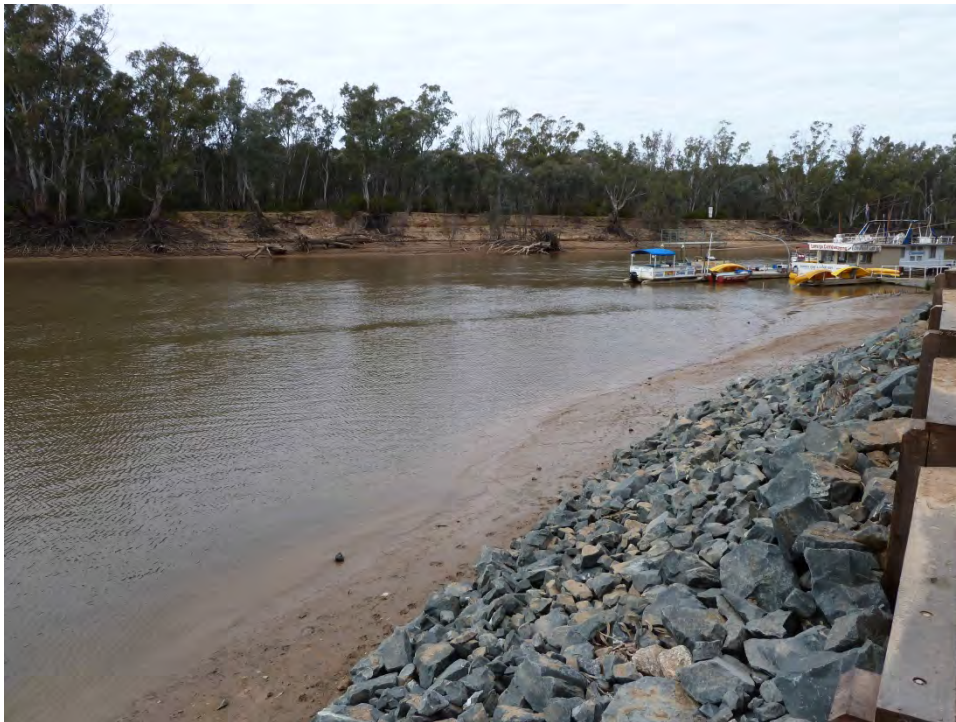
Figure 5 Murray River at proposed bridge crossing - Victorian bank; facing upstream (top) and downstream (bottom). Rock beaching placed along bank on either side of boat ramp
