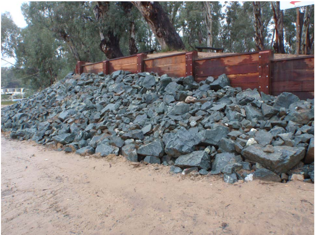
Photo 27 – Recent scour protection works at proposed Murray River crossing (2014)
