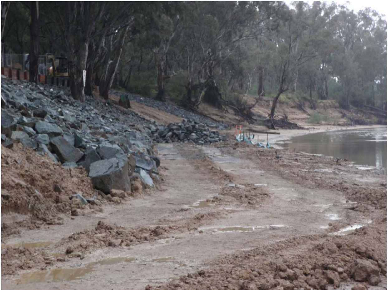
Photo 26 – Recent scour protection works at proposed Murray River crossing (2014)
