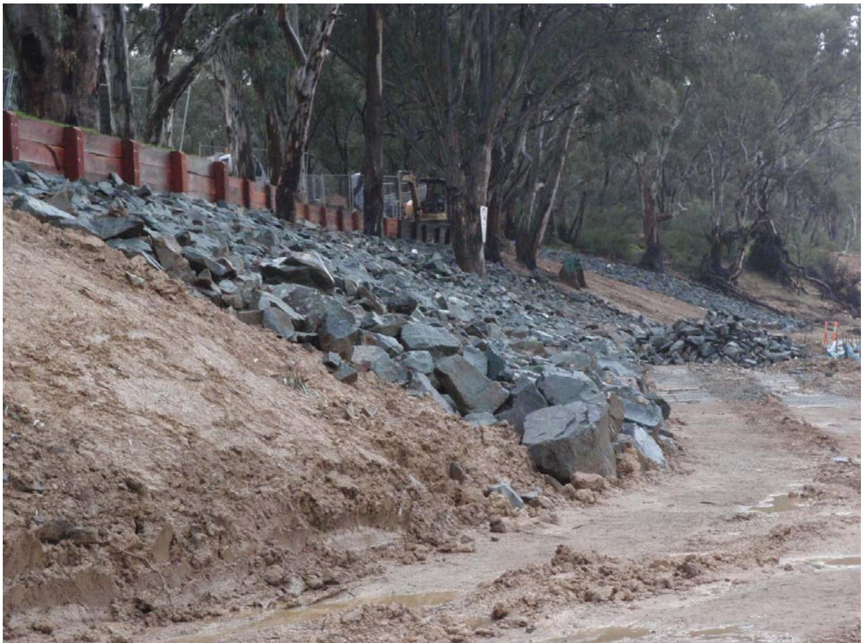
Photo 25 – Recent scour protection works at proposed Murray River crossing (2014)
