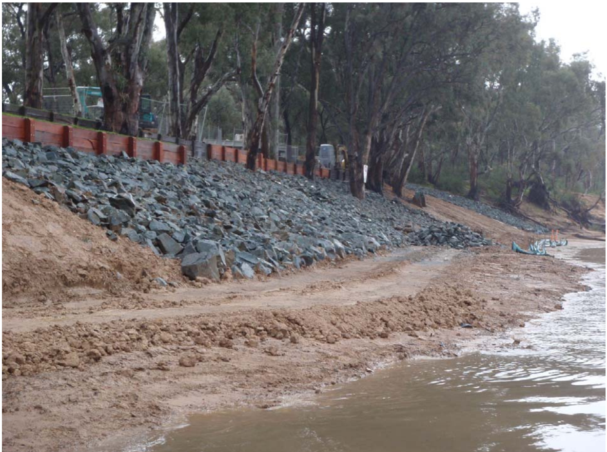
Photo 29 – Recent scour protection works at proposed Murray River crossing (2014)
