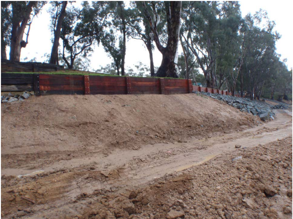
Photo 24 – Recent scour protection works at proposed Murray River crossing (2014)
