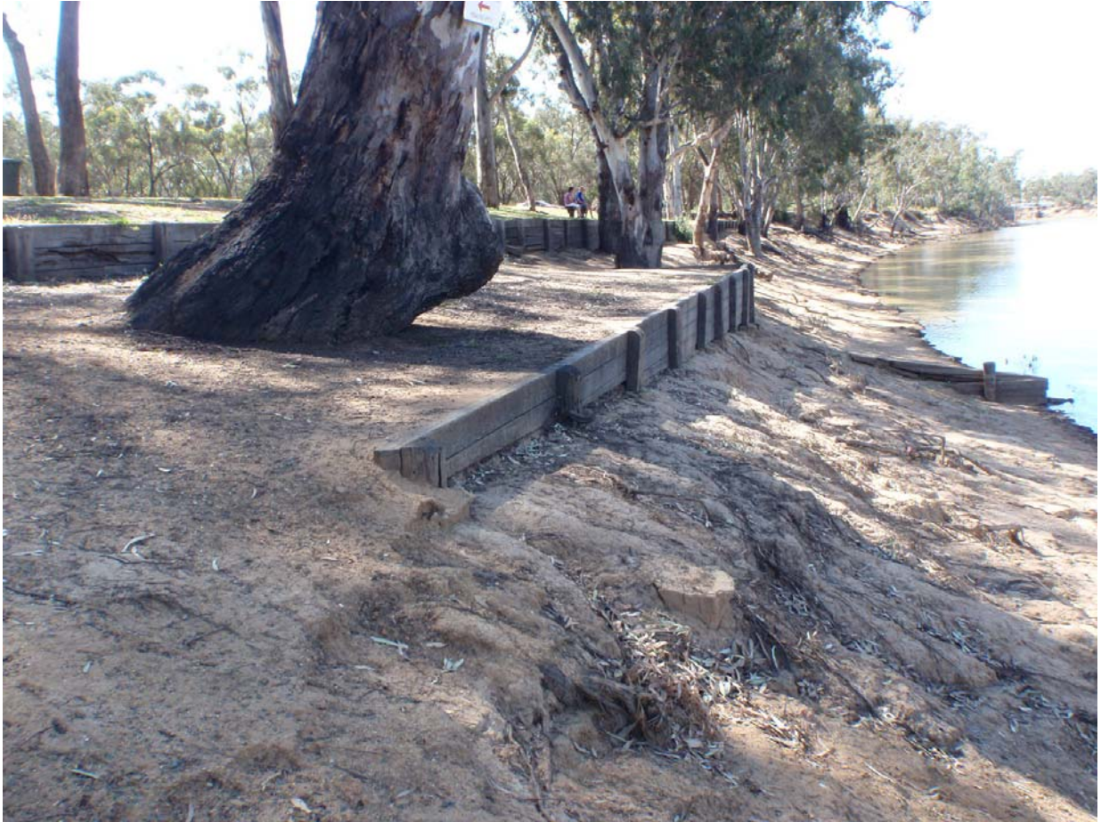
Photo 18 - Adjacent to boat ramp existing wooden retaining walls for scour protection (2011)
