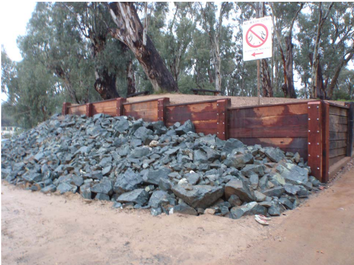
Photo 23 – Recent scour protection works at proposed Murray River crossing (2014)
