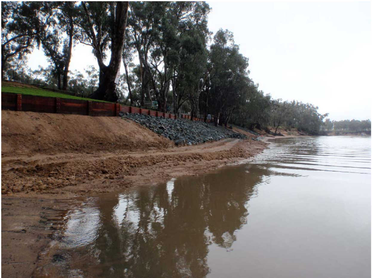
Photo 28 – Recent scour protection works at proposed Murray River crossing (2014)
