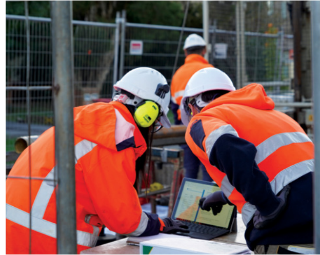
SRL East site investigations at Glen Waverley
