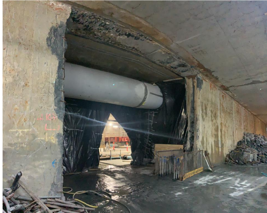
D-Wall Demolition in the Tram Box
