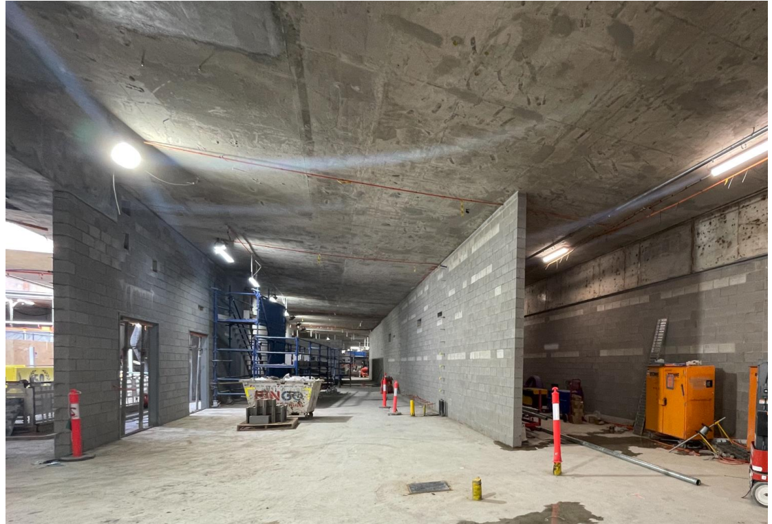
South box concourse level construction
