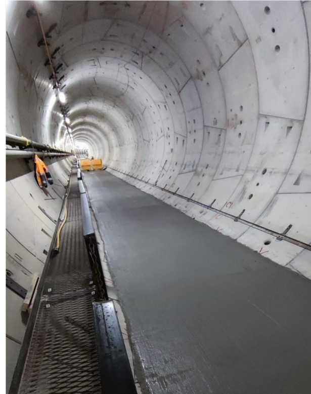
Tunnel invert works towards Eastern Portal
