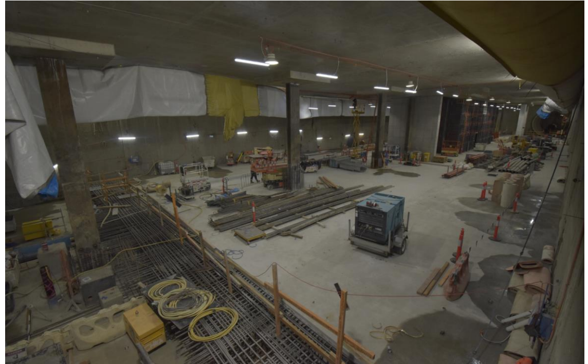
Base slab construction continues
