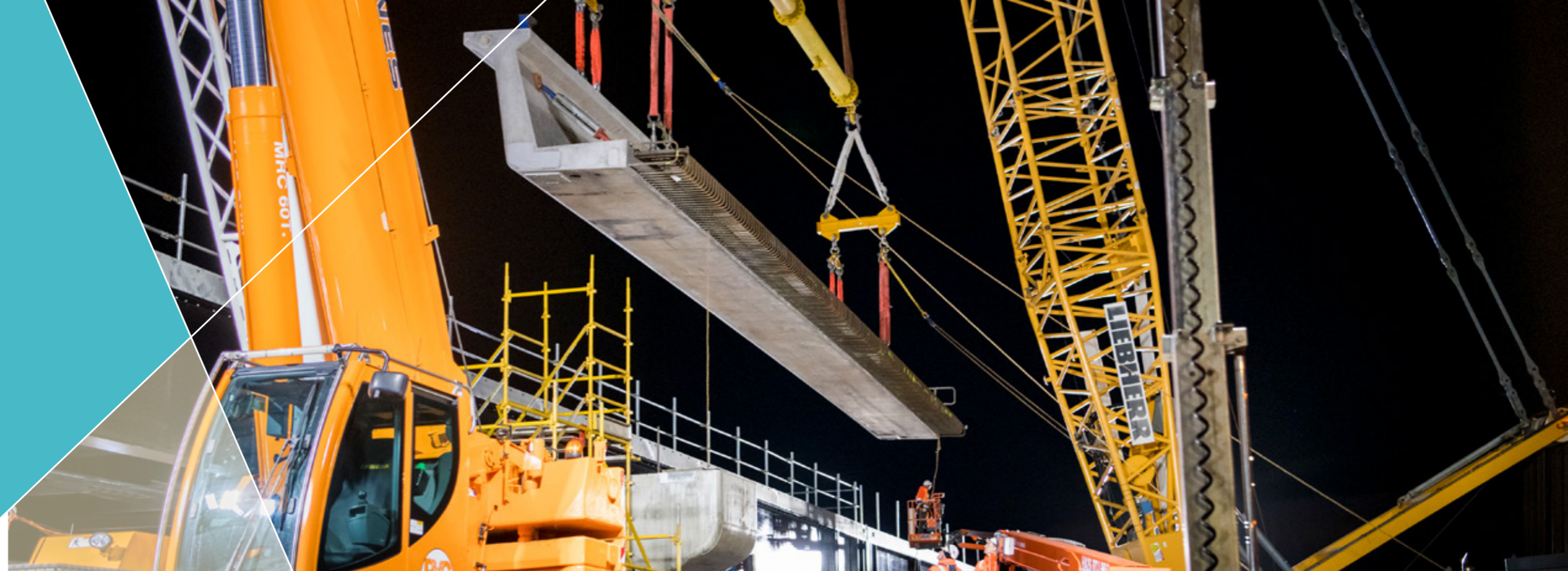
L-Beam installation on the Reservoir Level Crossing Removal Project
