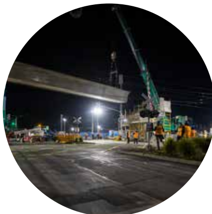
L beams being lifted into place by crane at Manchester Road
