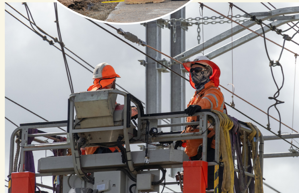
Works underway on overhead powerlines
