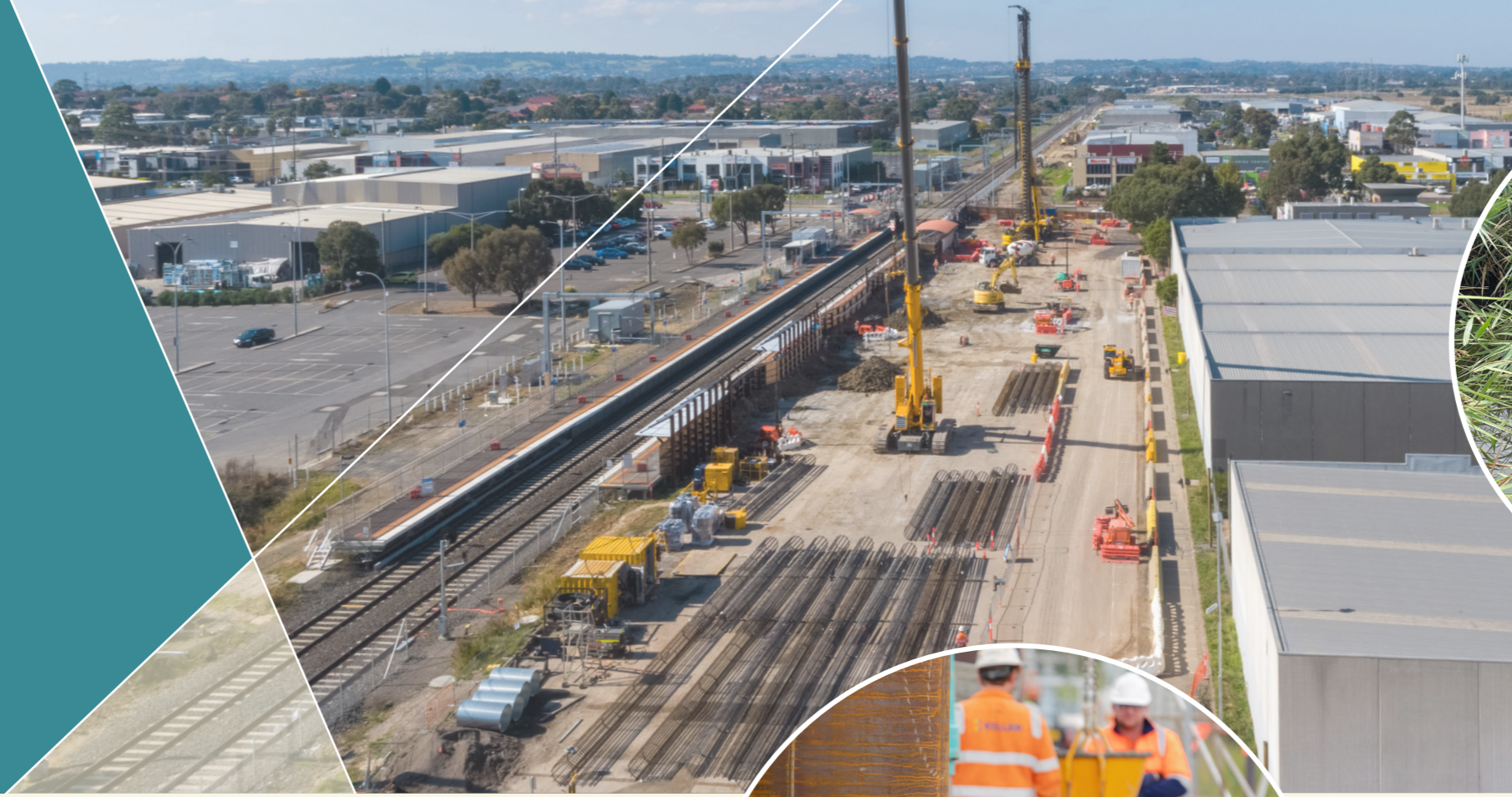
Foundation works for new rail bridge and station at Hallam
