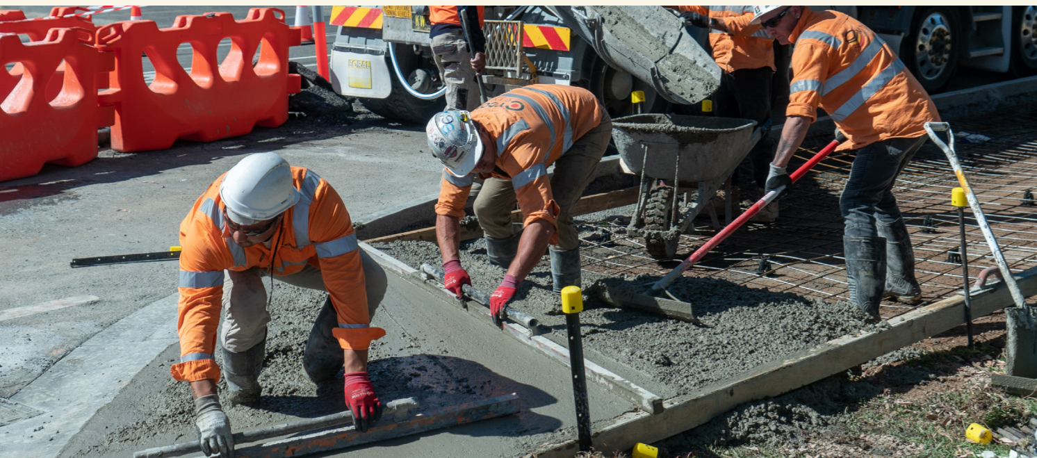
Crews lay foundations for new bus stop
