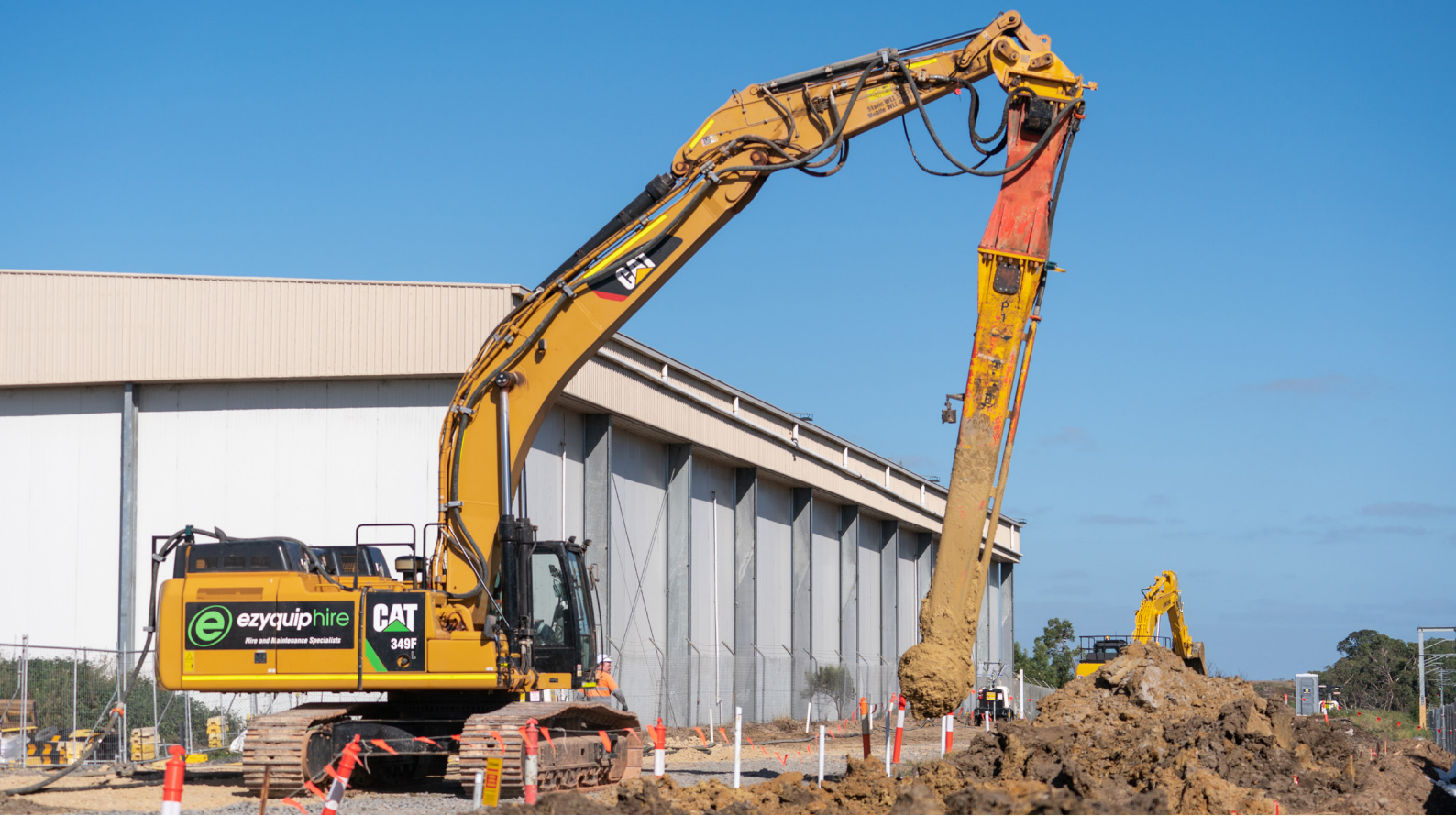
An excavator with rotating cutter attached for mass soil mixing
