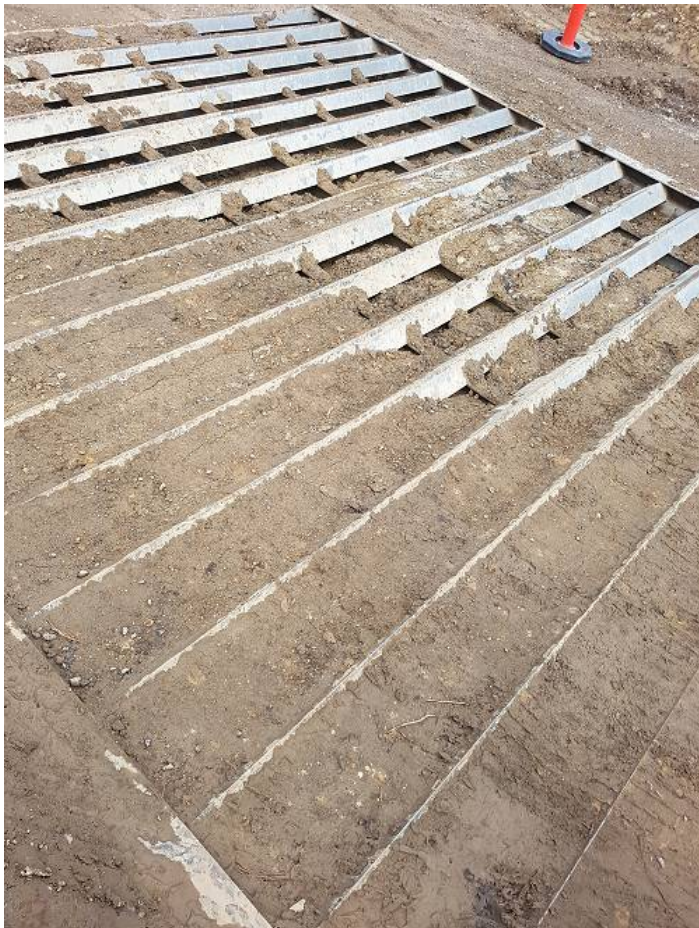
Left: The rumble grid located at the Centre Dandenong Road works exit required cleaning.
