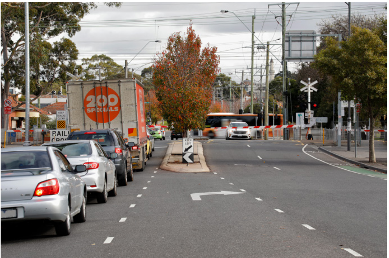
Cramer Street level crossing
