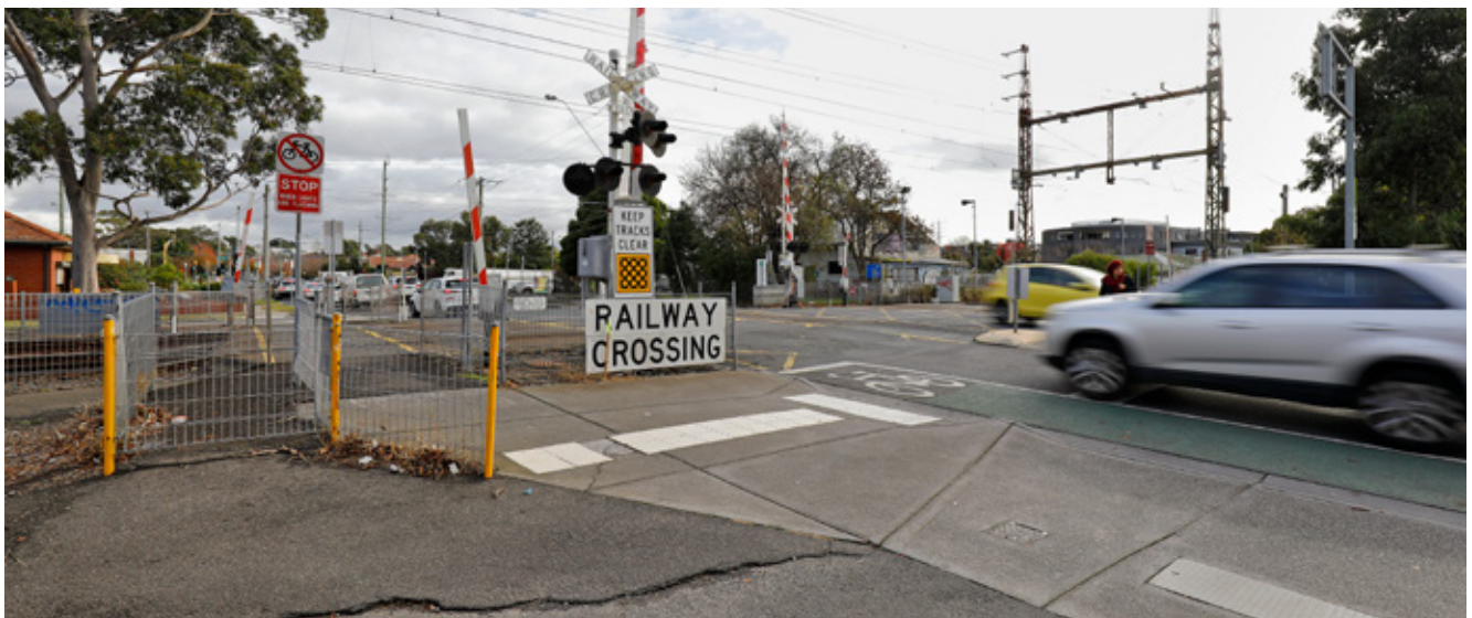
Cramer Street level crossing
