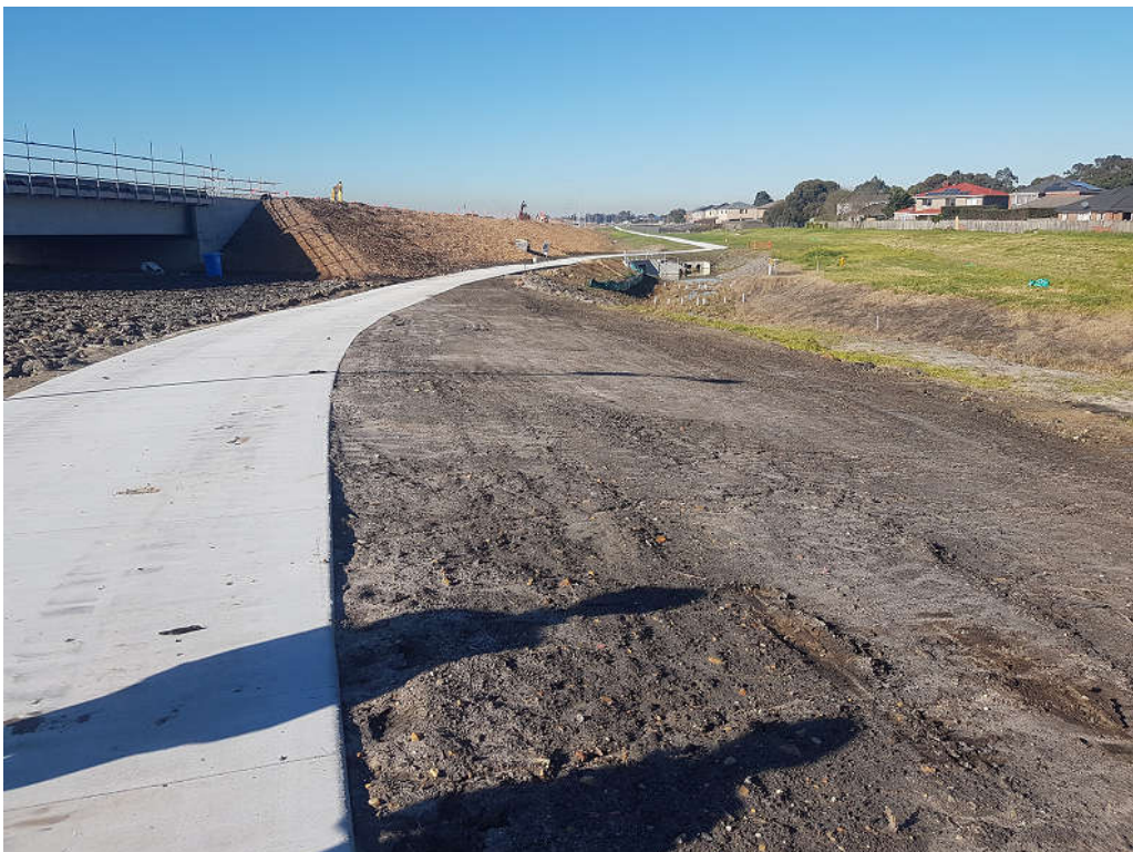
Above: New public pathway in Waterway area. Landscaping in progress.
