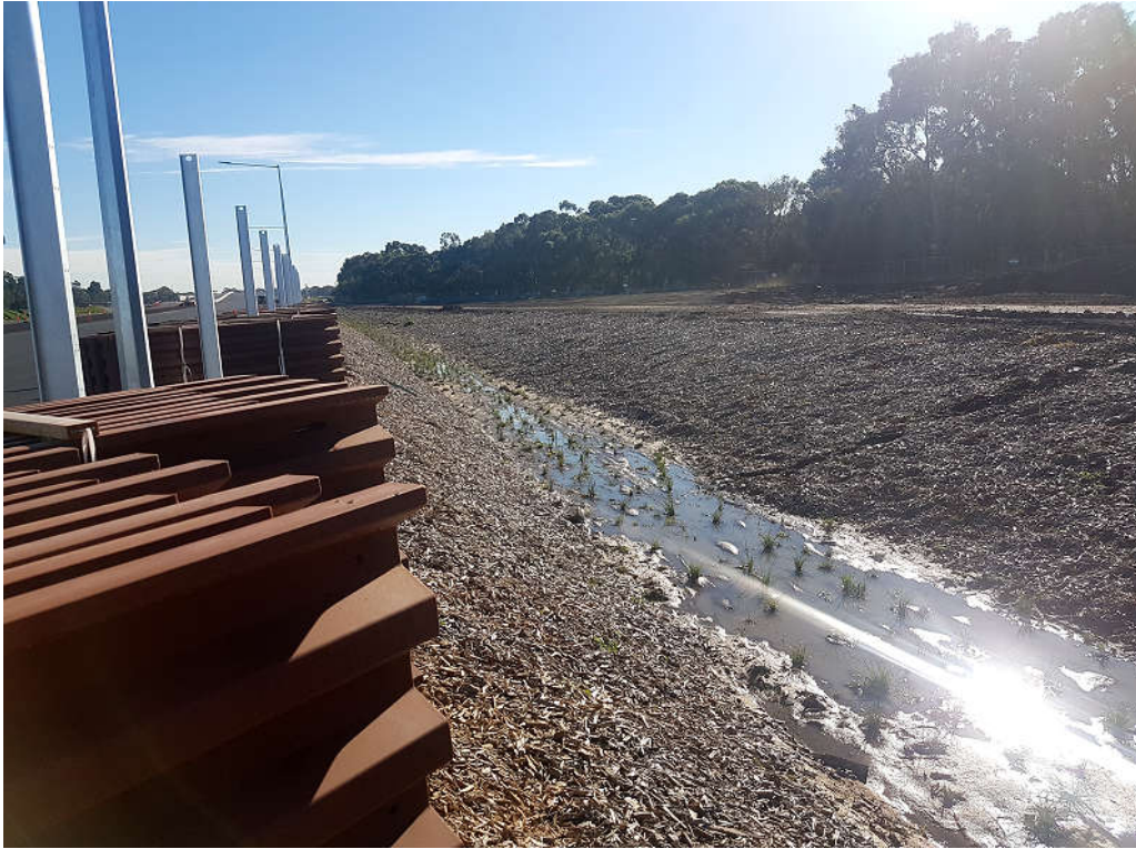
Above: Completed swale drain with screening panels awaiting installation.
