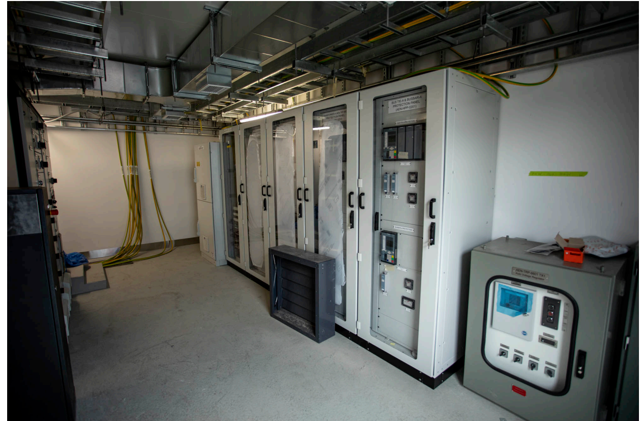
Internal equipment at ISS
