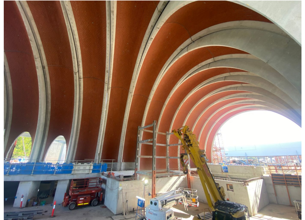
Arden Station entrance arches
