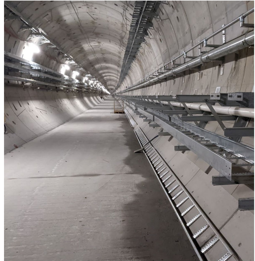
Rail tunnel fitout progress – Arden to Parkville
