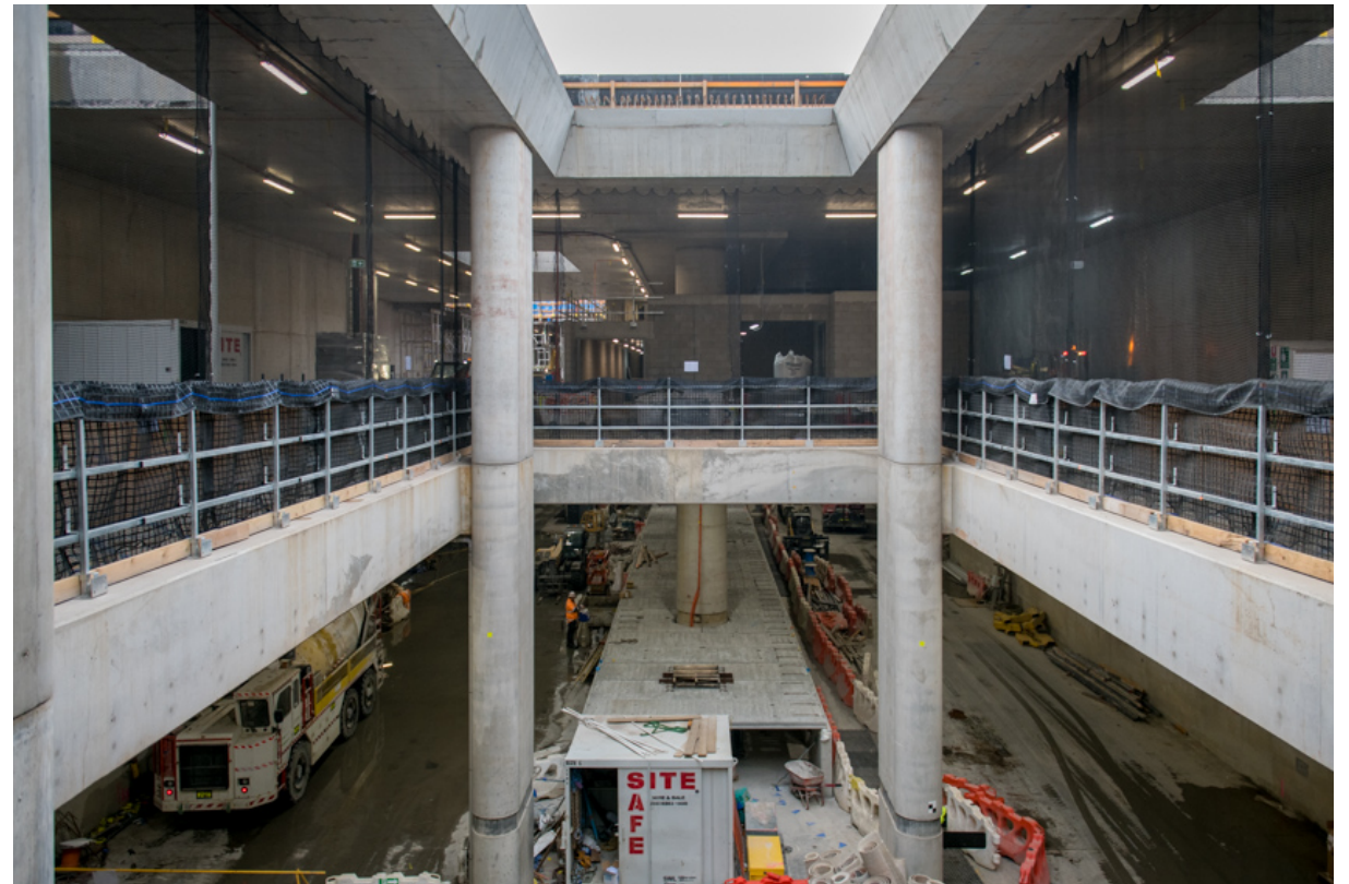
Platform construction progress – prior to completion
