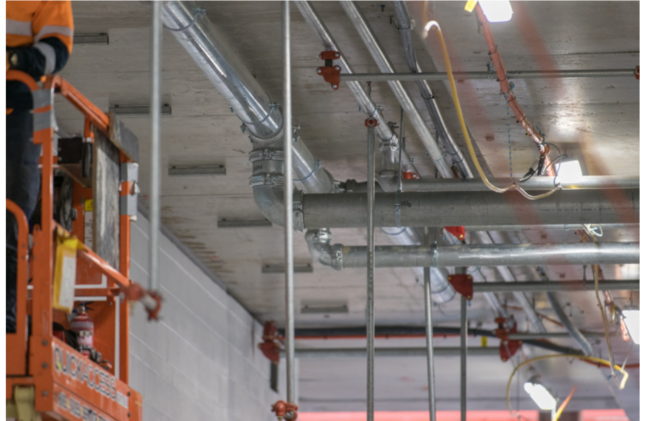
Mechanical, electrical and plumbing rough-in – service building
