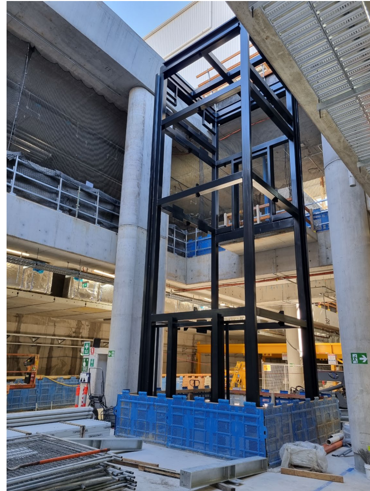
Lift shaft installation
