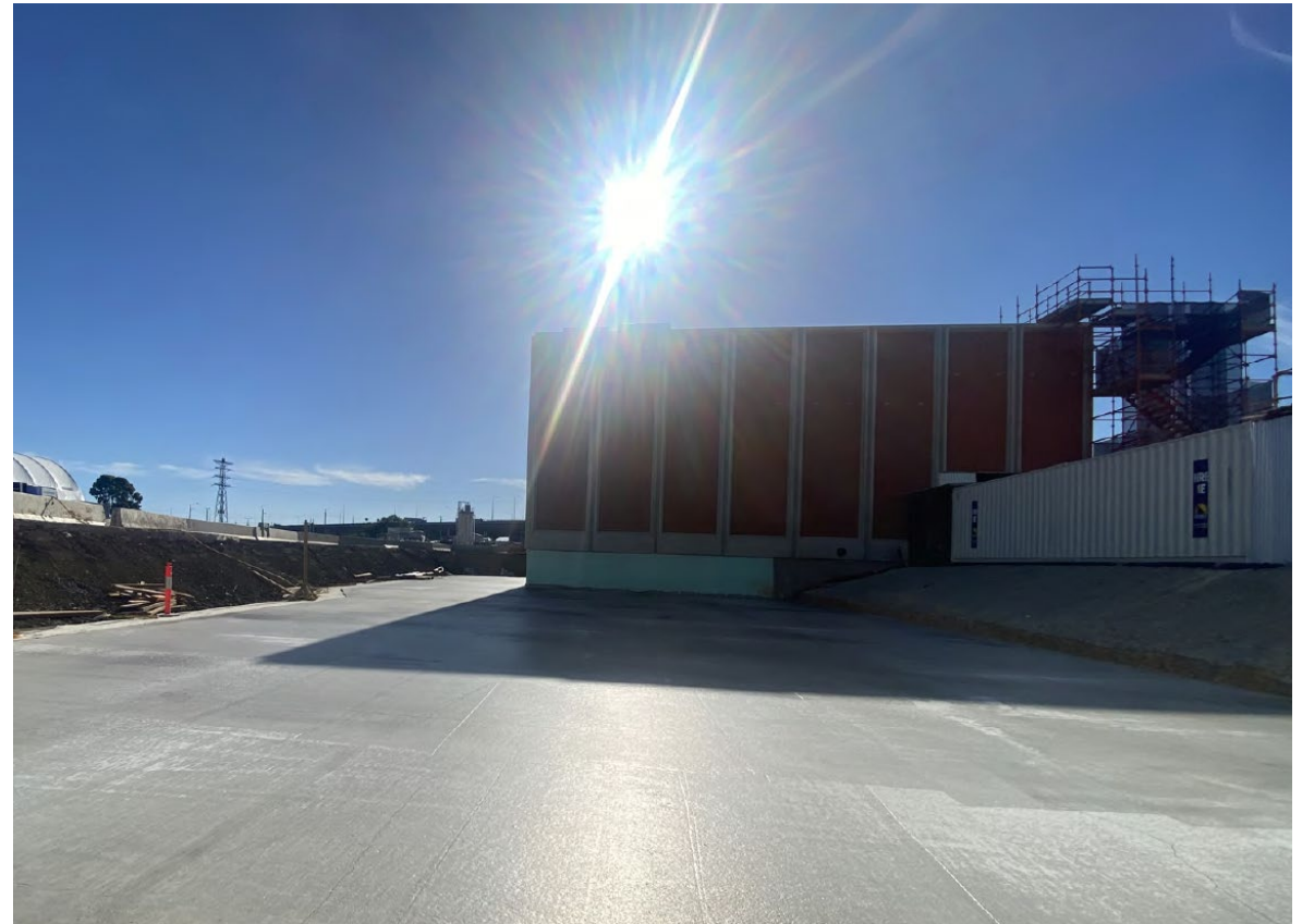
Waterproofing slab around the service building
