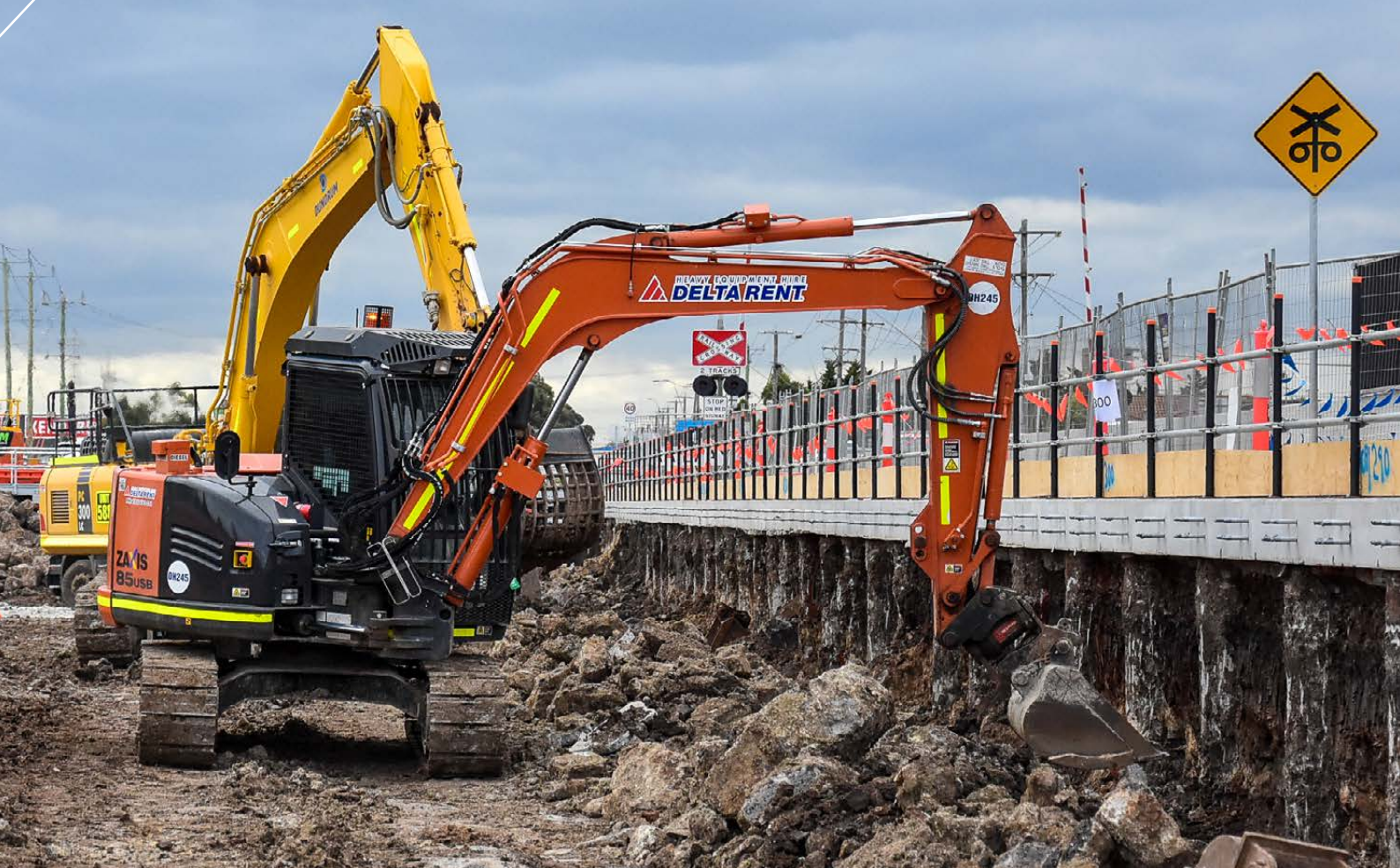
Earthworks are now progressing at Robinsons Road.
