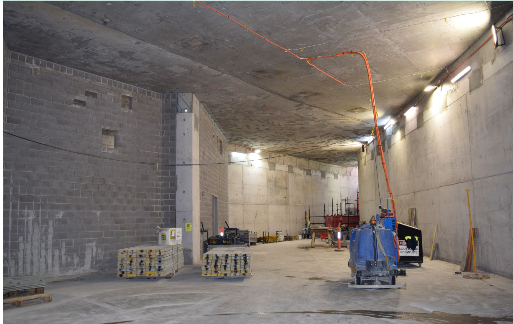
Blockwork wall install in the Grattan Street West station entrances
