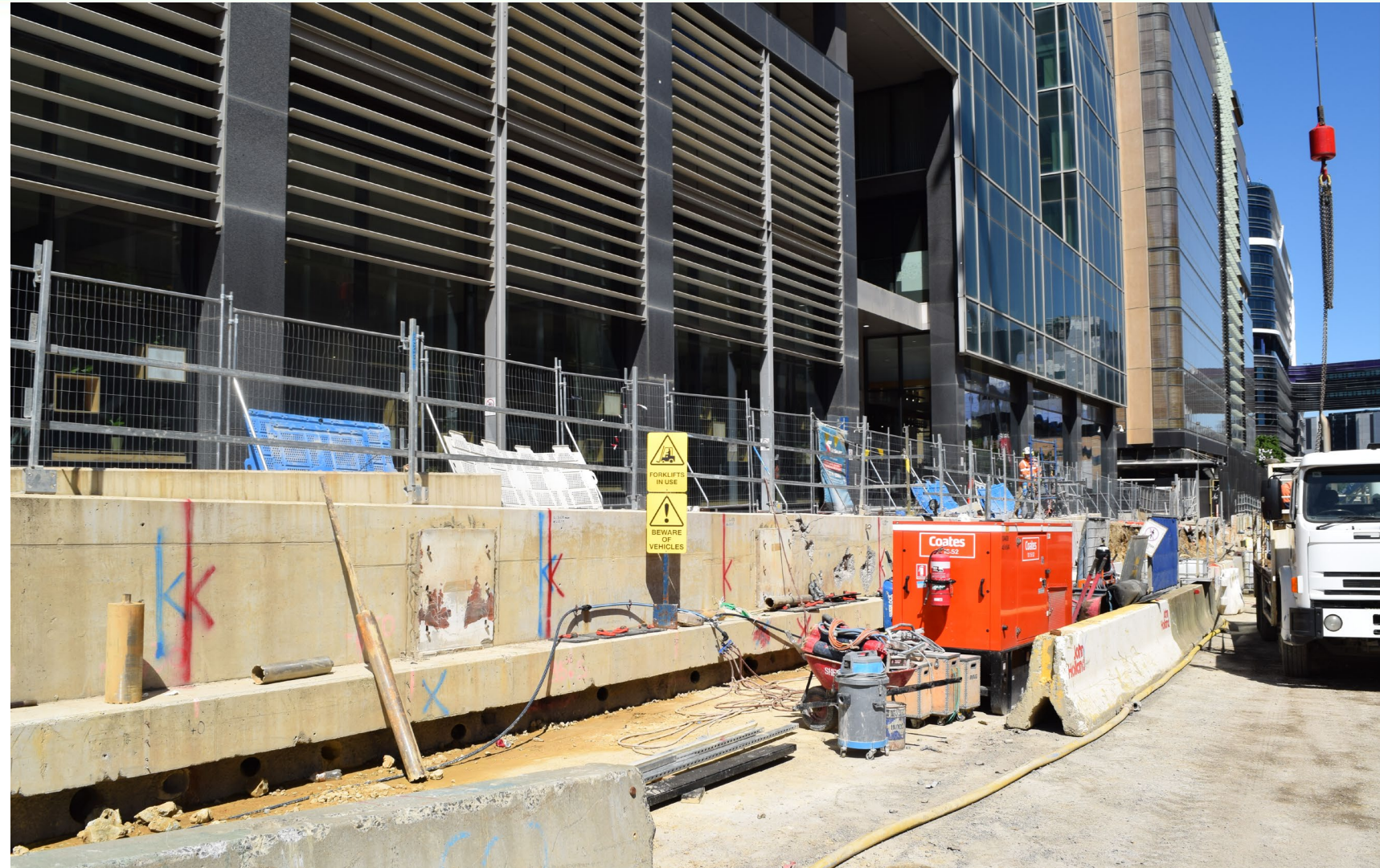
Berkeley to Barry street capping beam removal works
