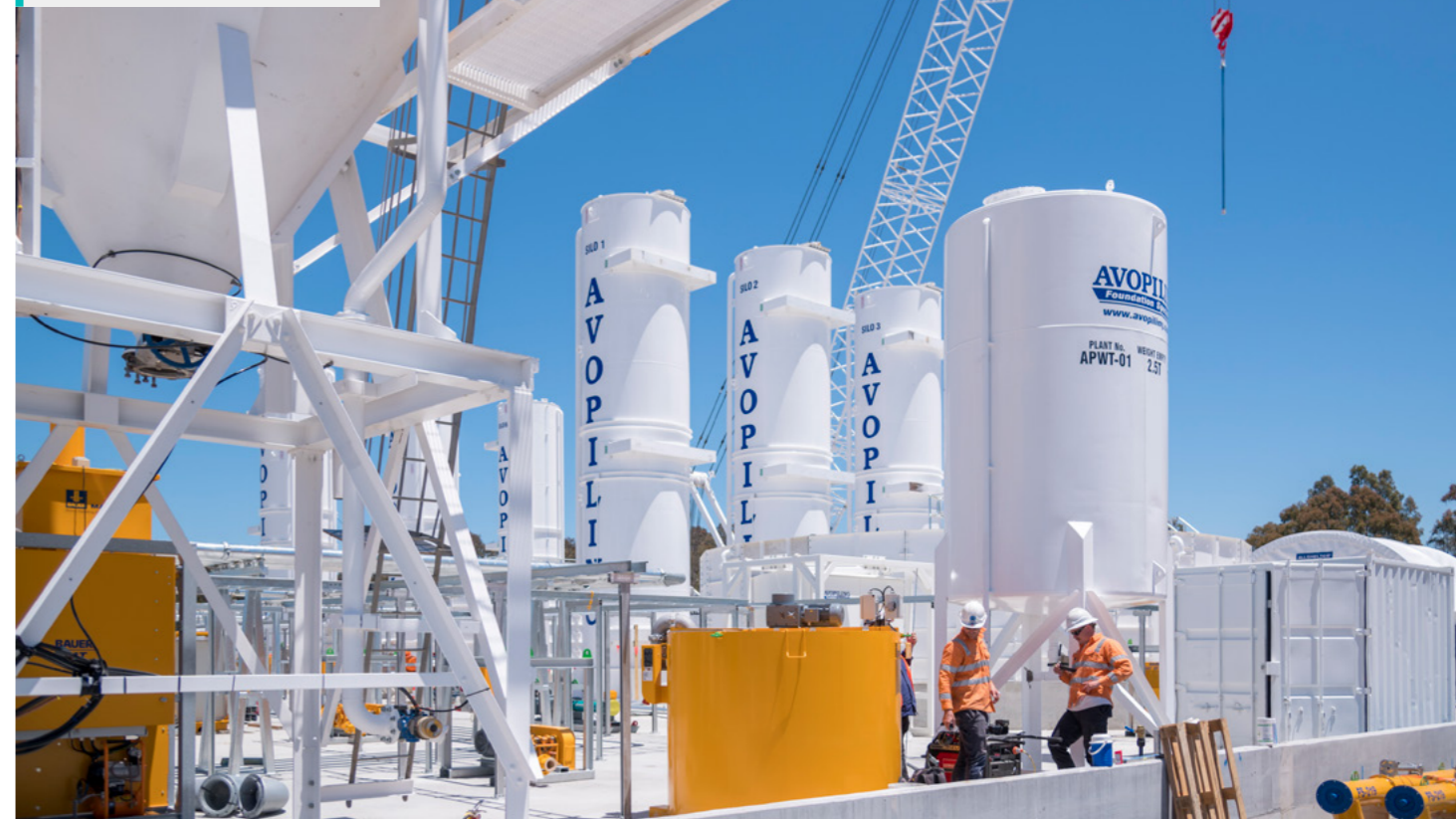
Clay manufacturing in operation at Greenaway Street worksite
