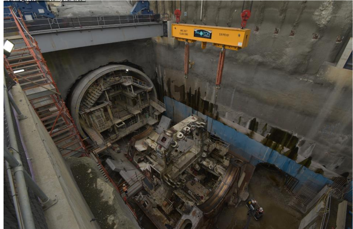
The main drive waiting to be lifted
