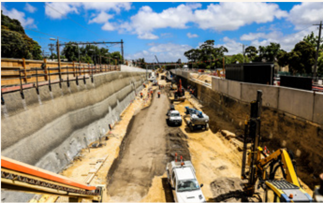
Construction of the lowered rail cutting (Carroll Crescent)
