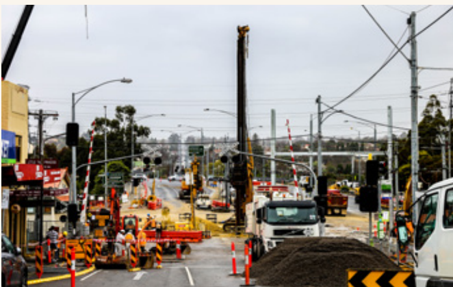
Construction of the Burke Road bridge deck
