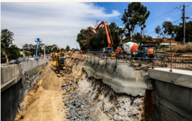
Construction of the lowered rail cutting (Wills Street)
