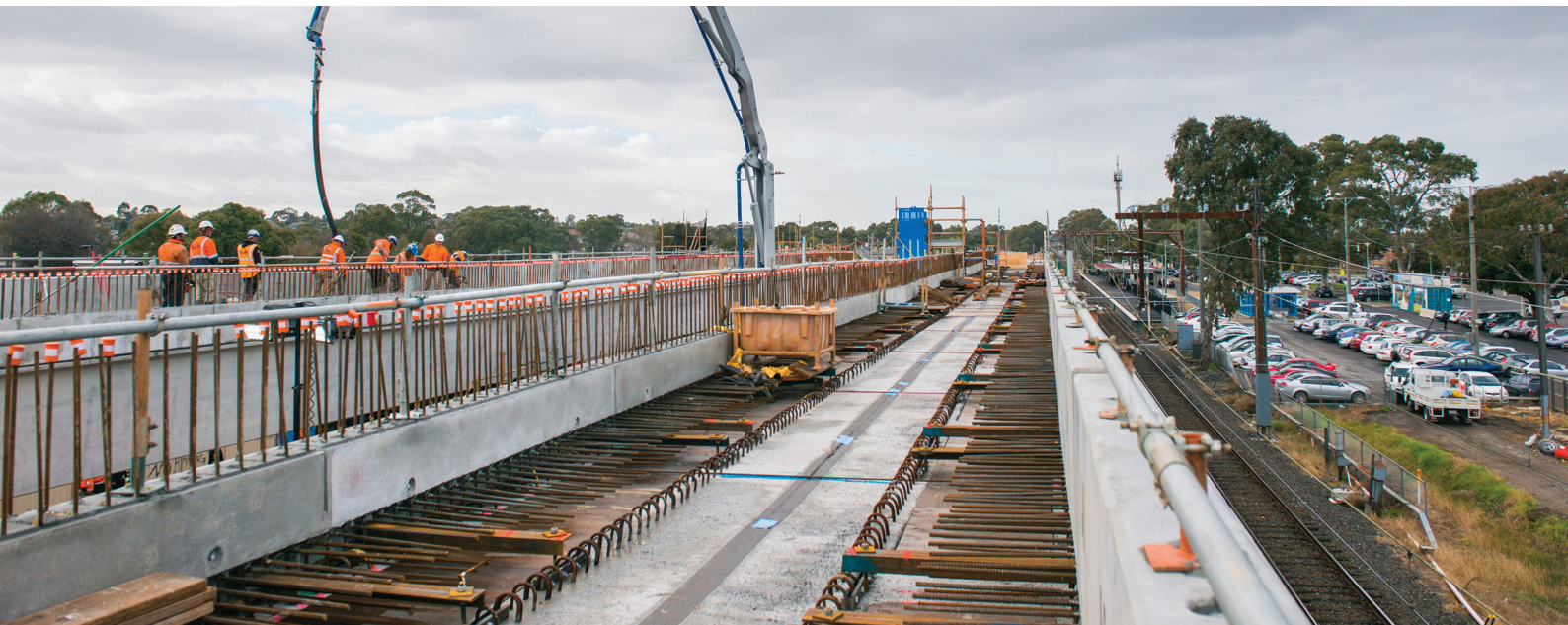
Pouring of the elevated deck, Noble Park Station.
