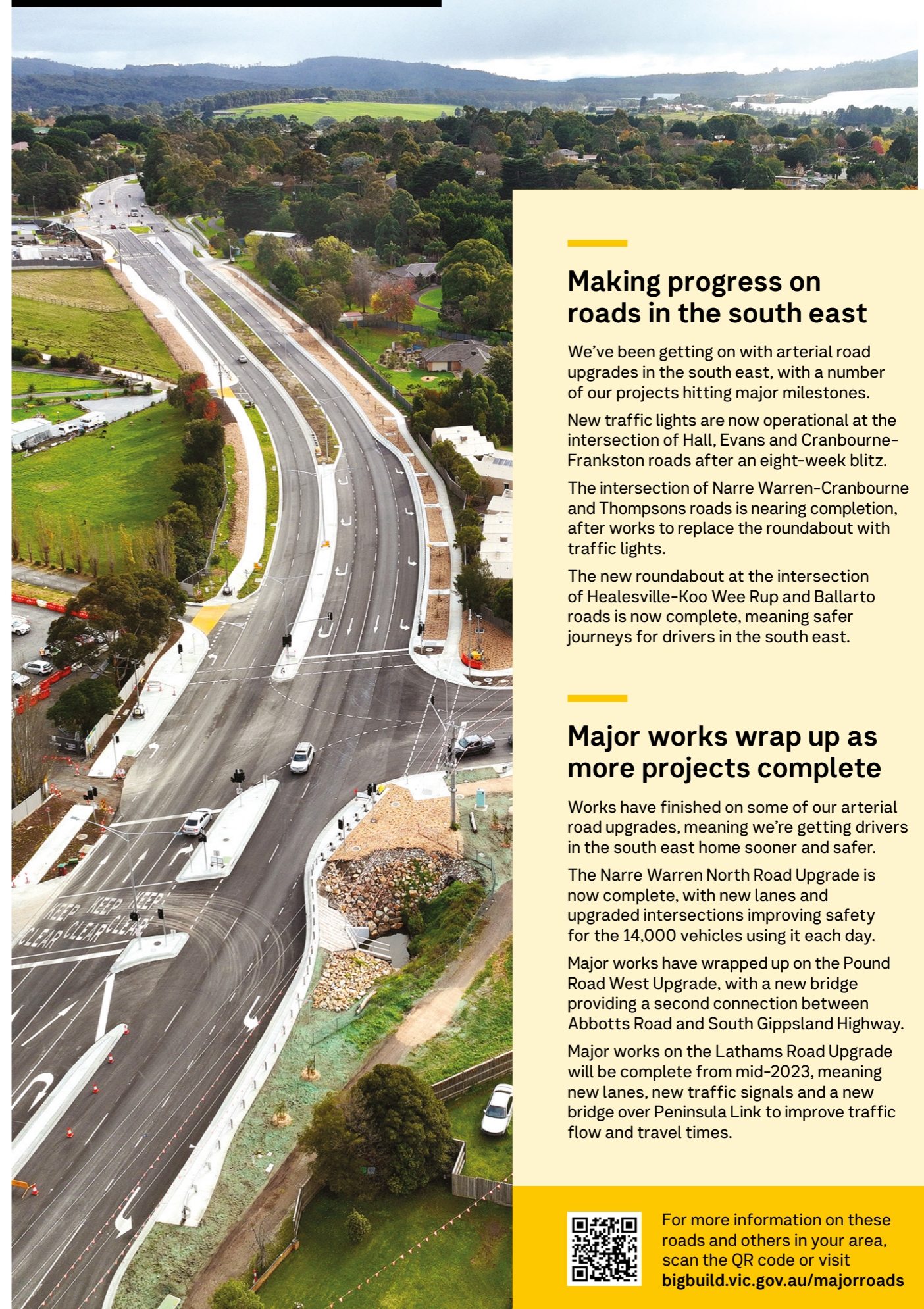
The recently completed Narre Warren North Road upgrade
