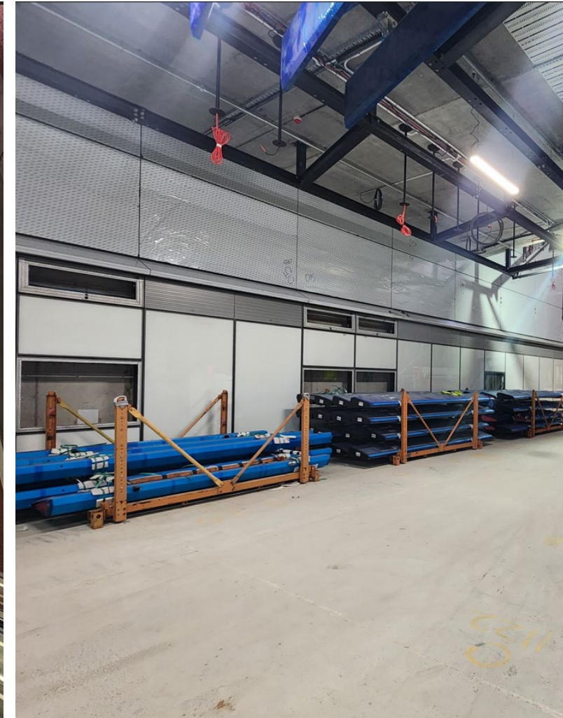
Installation of cladding above colour back glass
