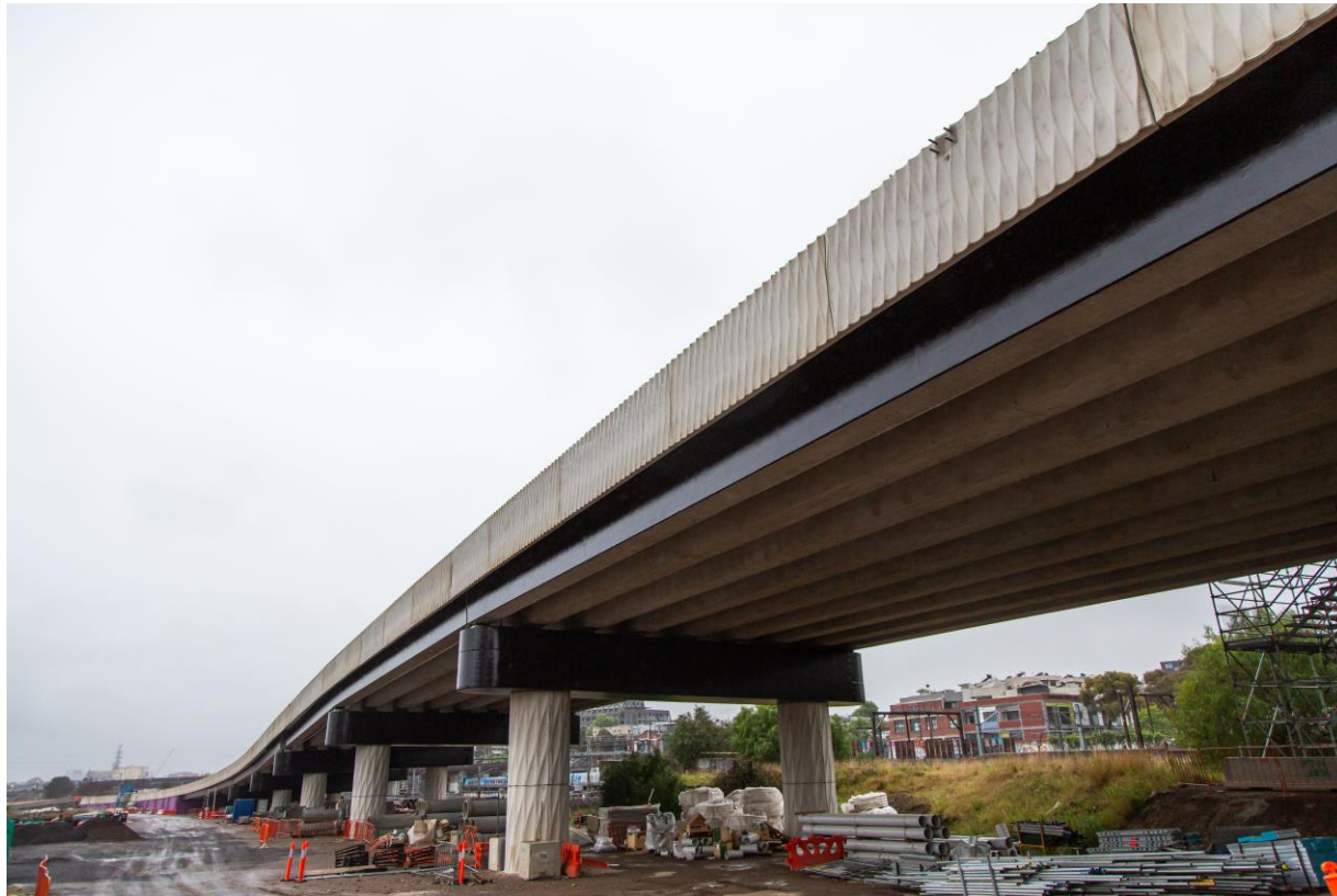
Wurundjeri Way Extension bridge
