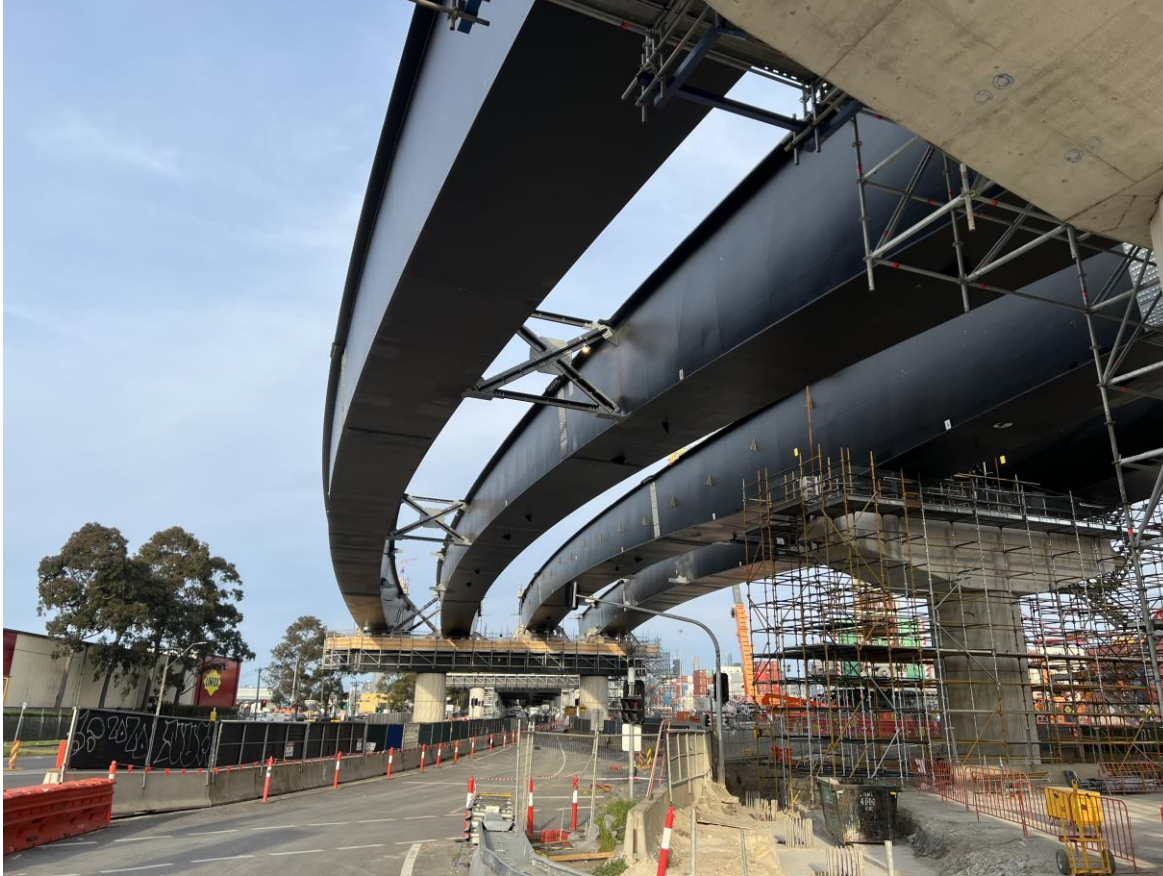
Final girders being lifted into place to connect elevated road to Maribyrnong River Bridges
