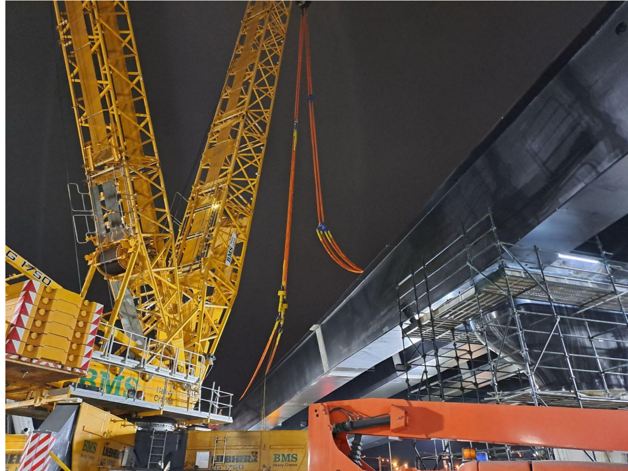
Final girder being lifted over Dynon Road
