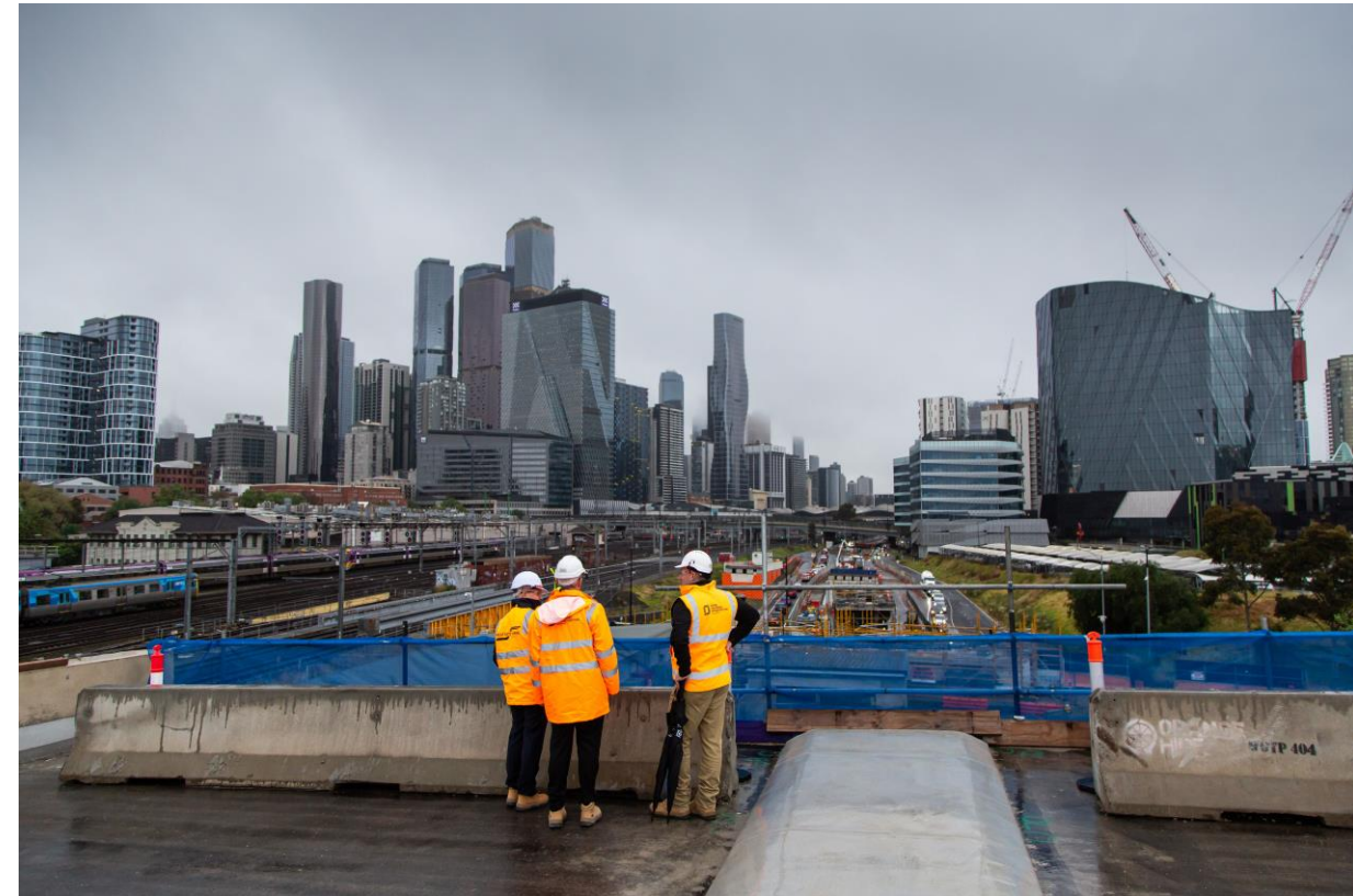
Overlooking Wurundjeri Way and Dudley Street Intersection
