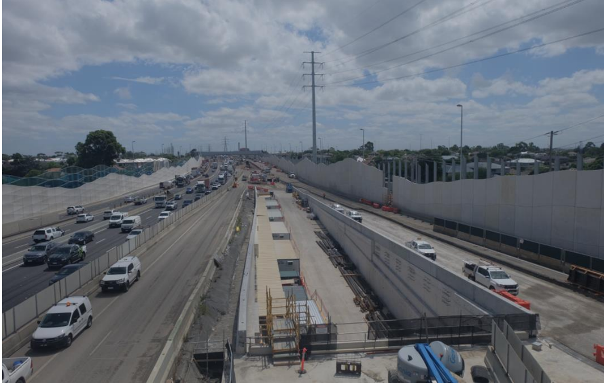
Southern tunnel entry preparing for construction of timber net structure
