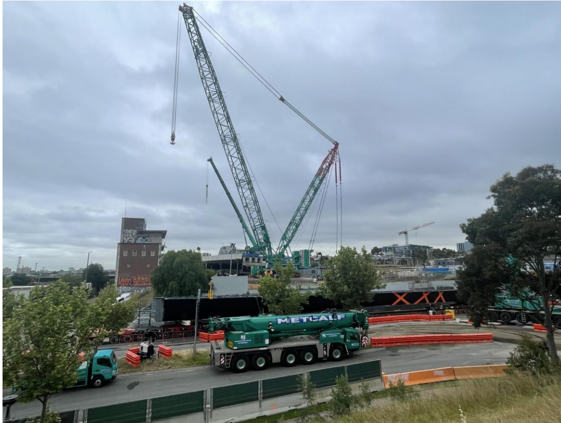
Beams being lifted into place over Dudley Street
