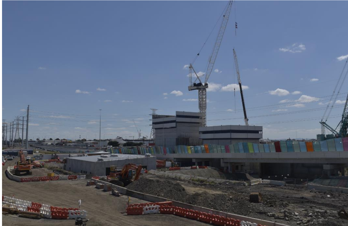
Southern tunnel exit ventilation structure currently 30m high
