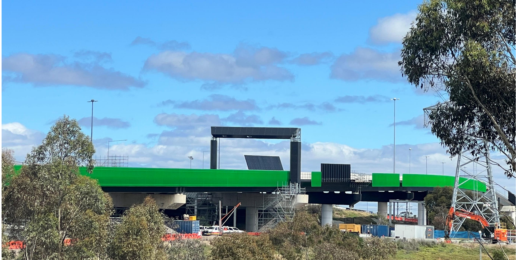
New gantry installed on Hyde Street inbound off ramp
