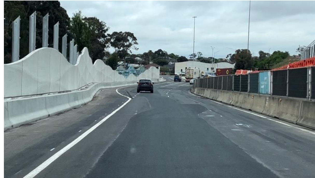
New second left hand turn from Williamstown Road outbound off ramp
