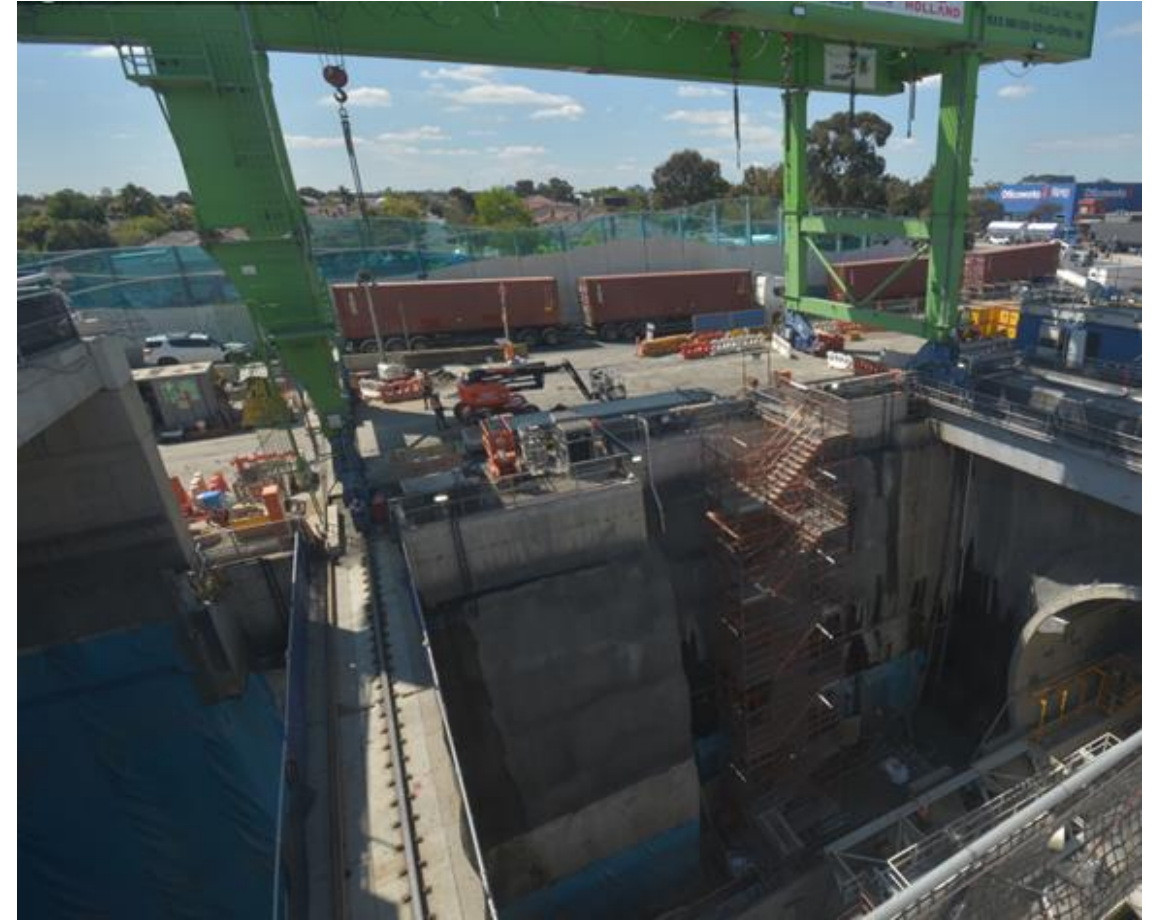
500 Tonne gantry crane soon to be demobilised
