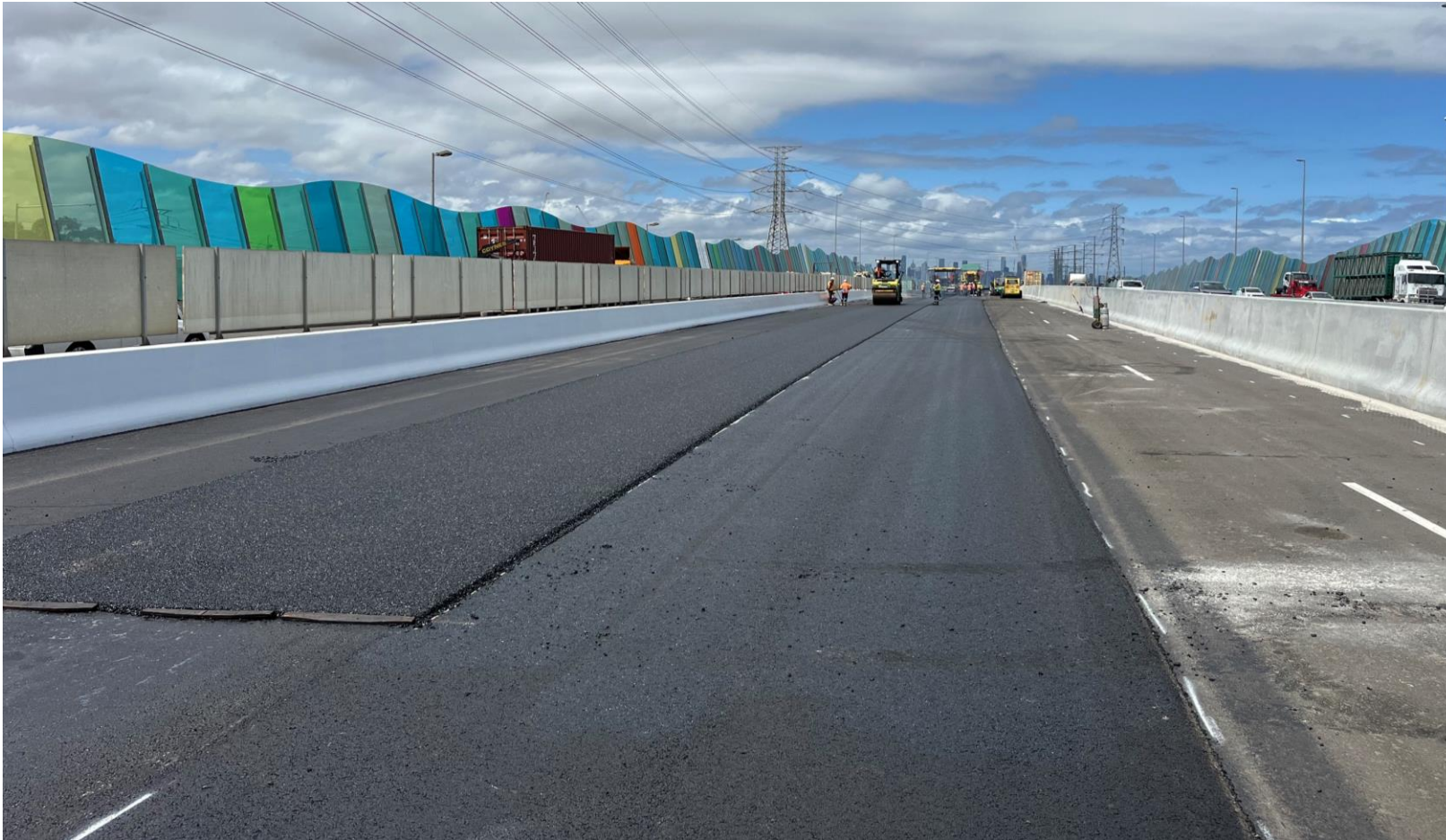
WGF Resurfacing – Facilitate Bridge Expansion Joint Works
