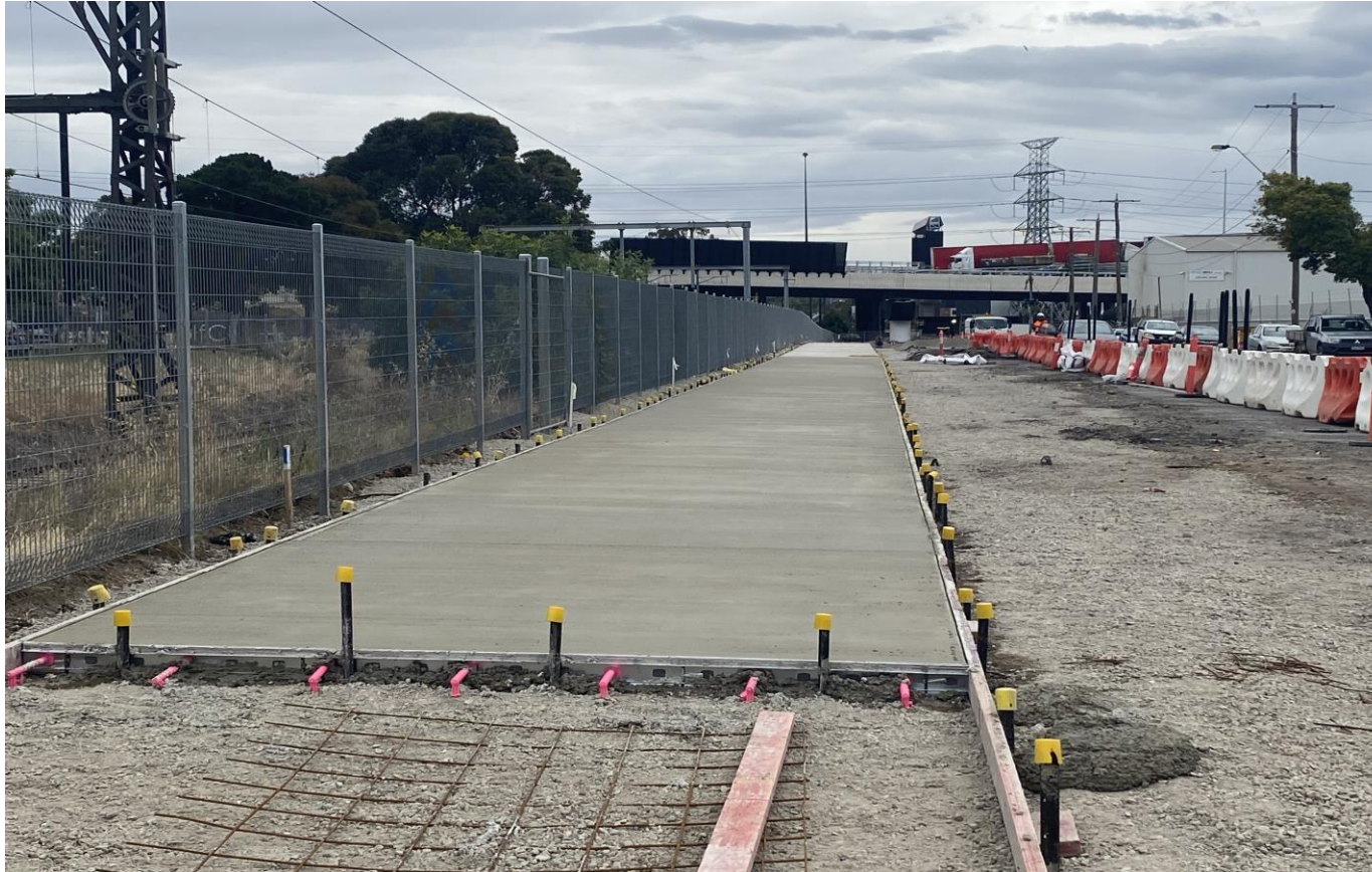
Preparations for Concrete Pour Hall Street between Simcock Ave and Freeway
