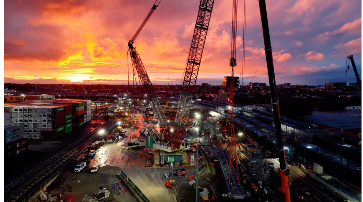
Final girders lifted into place on Footscray Road
