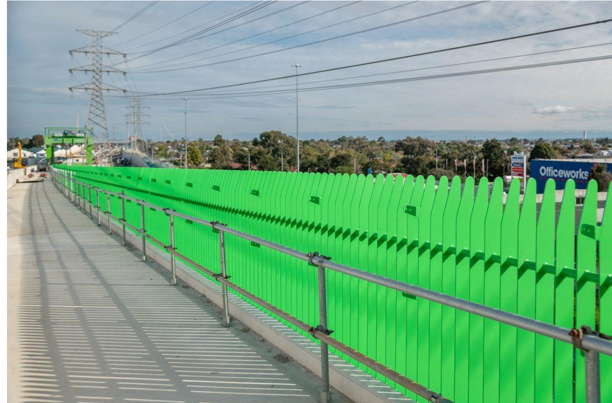
Shared walking and cycling path under construction
