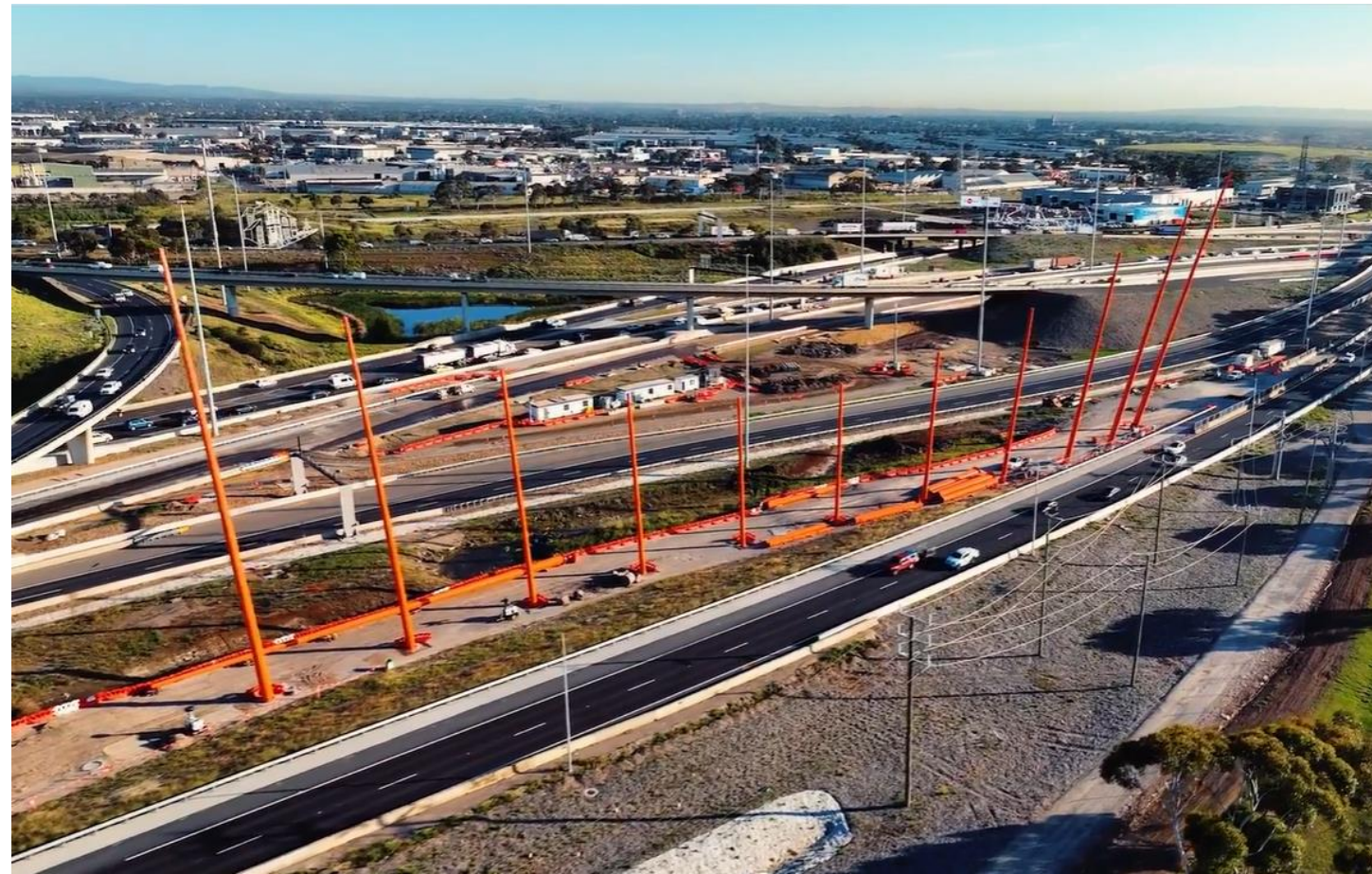
The M80 feature light poles have been installed
