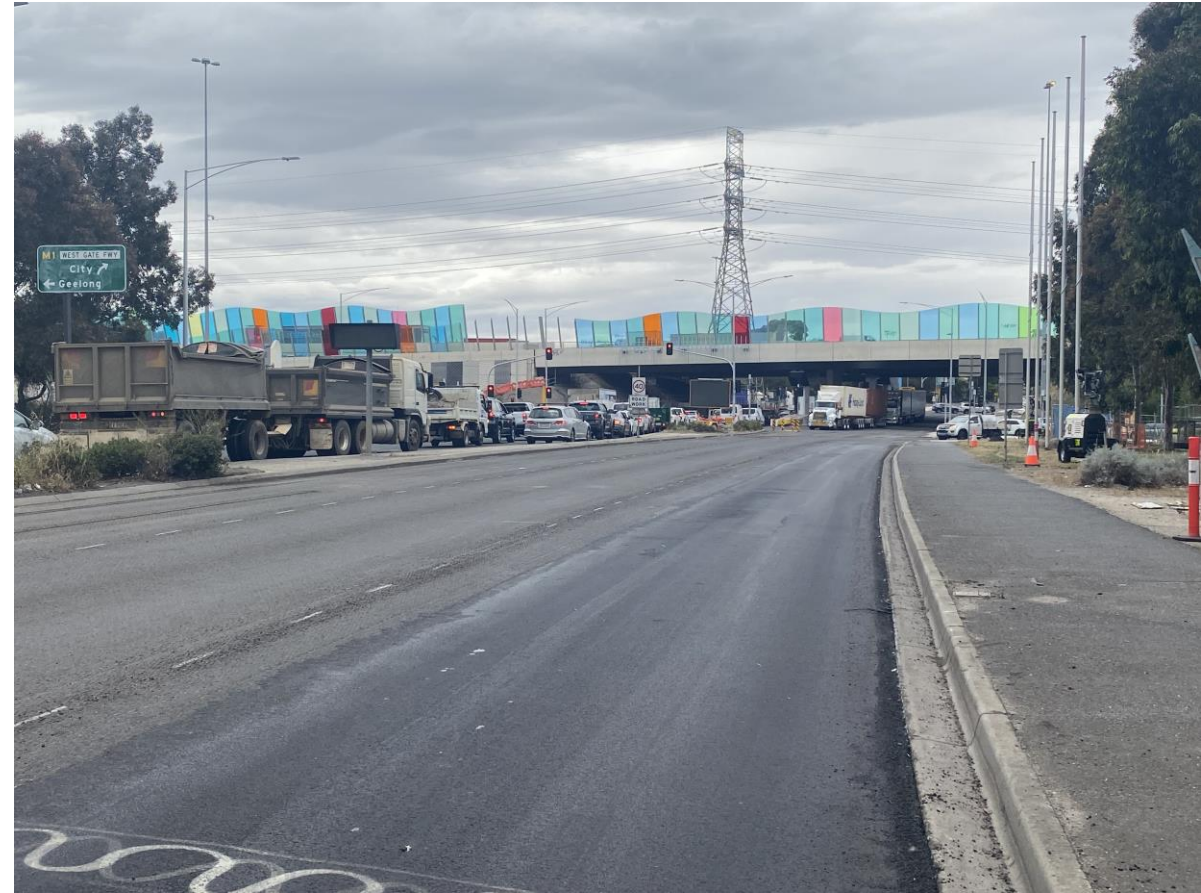
After – resurfacing underway
