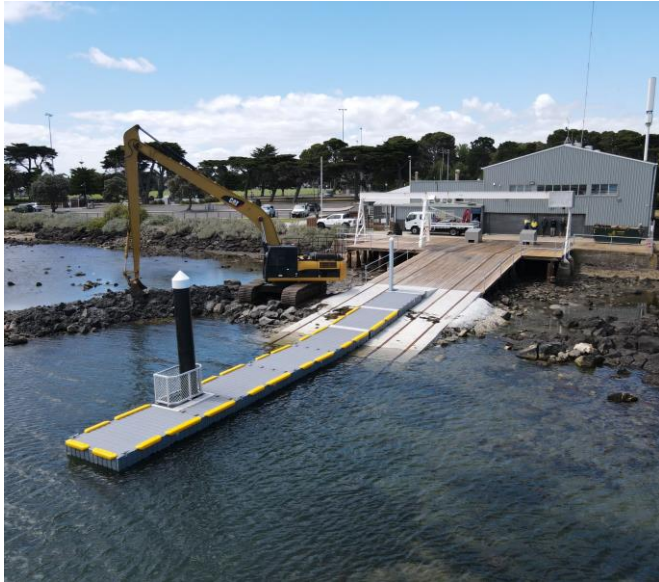
WGNF - Williamstown Jetty Refurbishment
