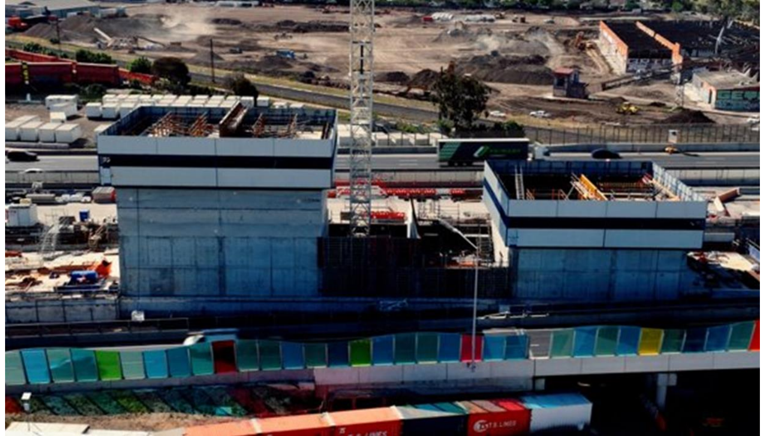
Progress of Southern Outbound Portal Vent Structure
