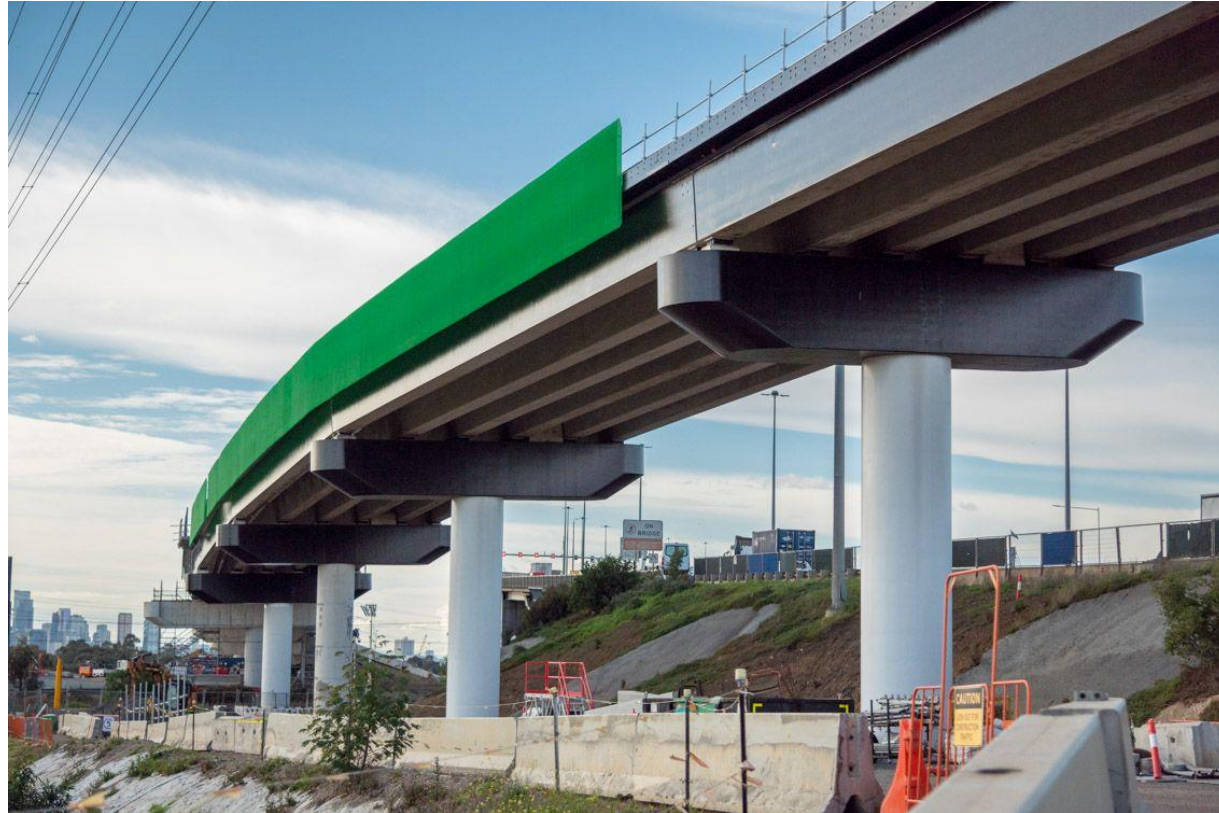
New inbound exit ramp to Hyde Street
