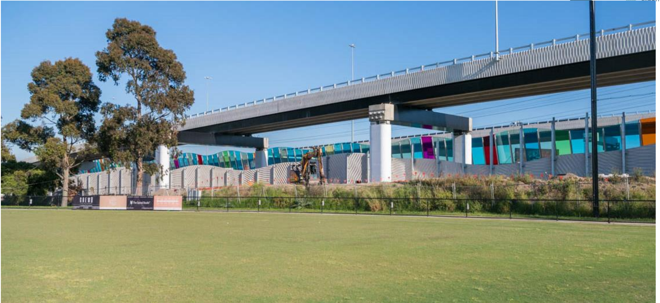
Noise wall panels – Acrylic panel installation is well underway
