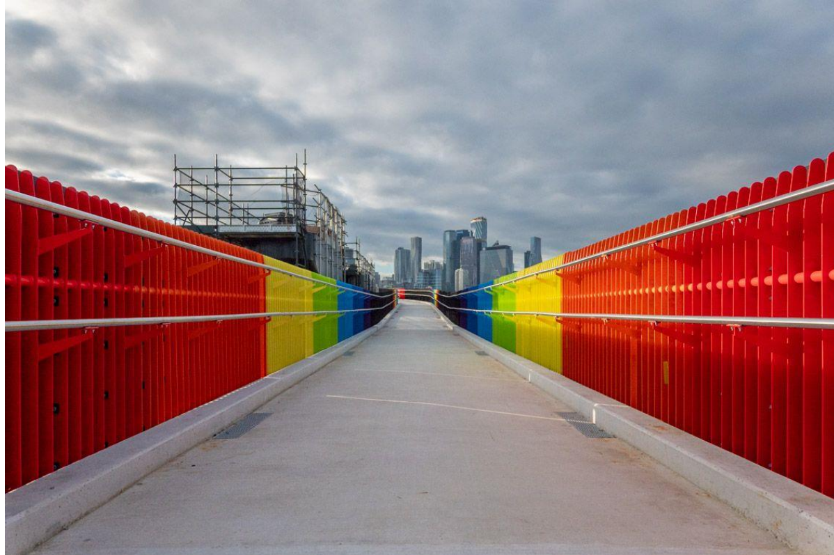
New Dynon Road SUP Bridge
