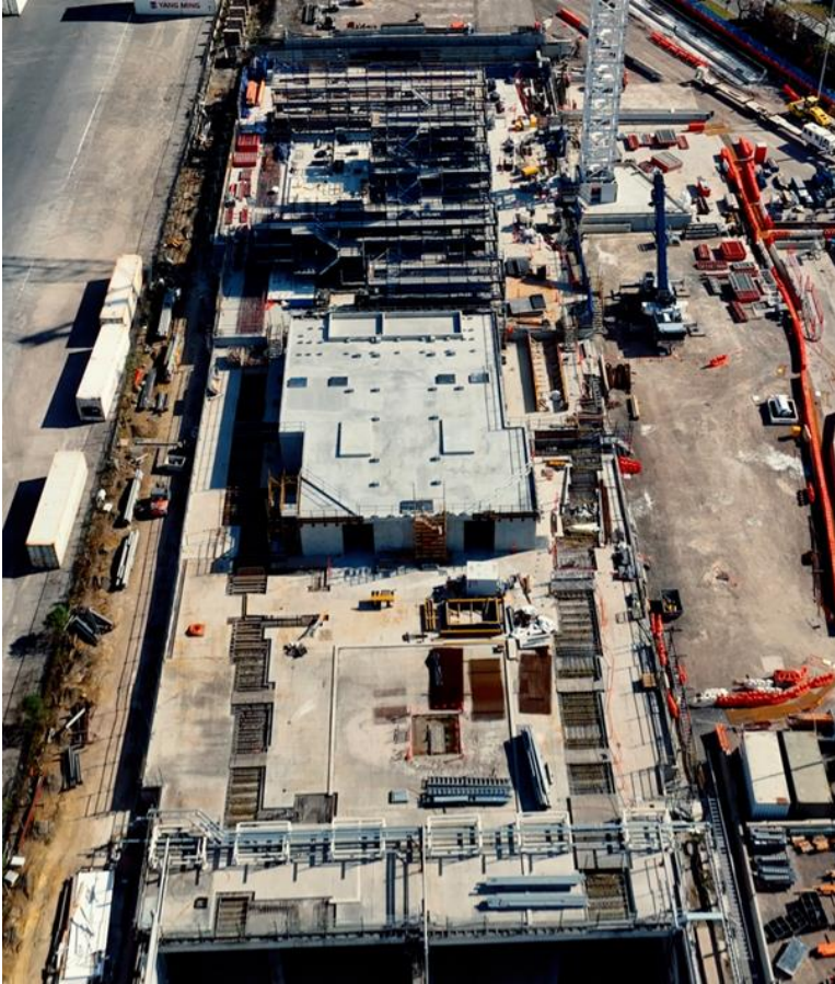
Progress of Northern Portal Vent Structure
