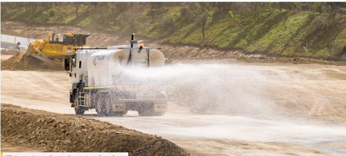
Water cart spraying work area to reduce dust
