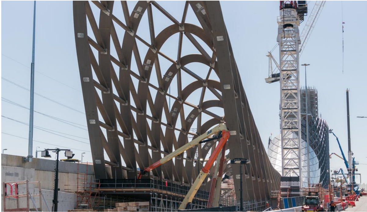
Southern Outbound exit diagrid structure and timber net installation progress
