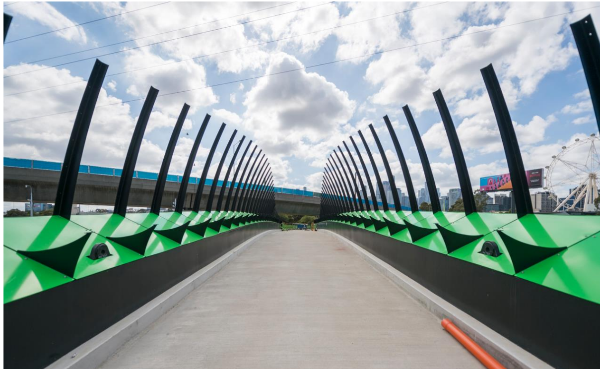
Eastern view of the Shared Use Path (SUP) bridge west of CityLink showing fin balustrades (mesh screening to be installed)
