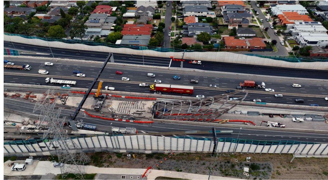
Southern Inbound tunnel entry with timber net structure
