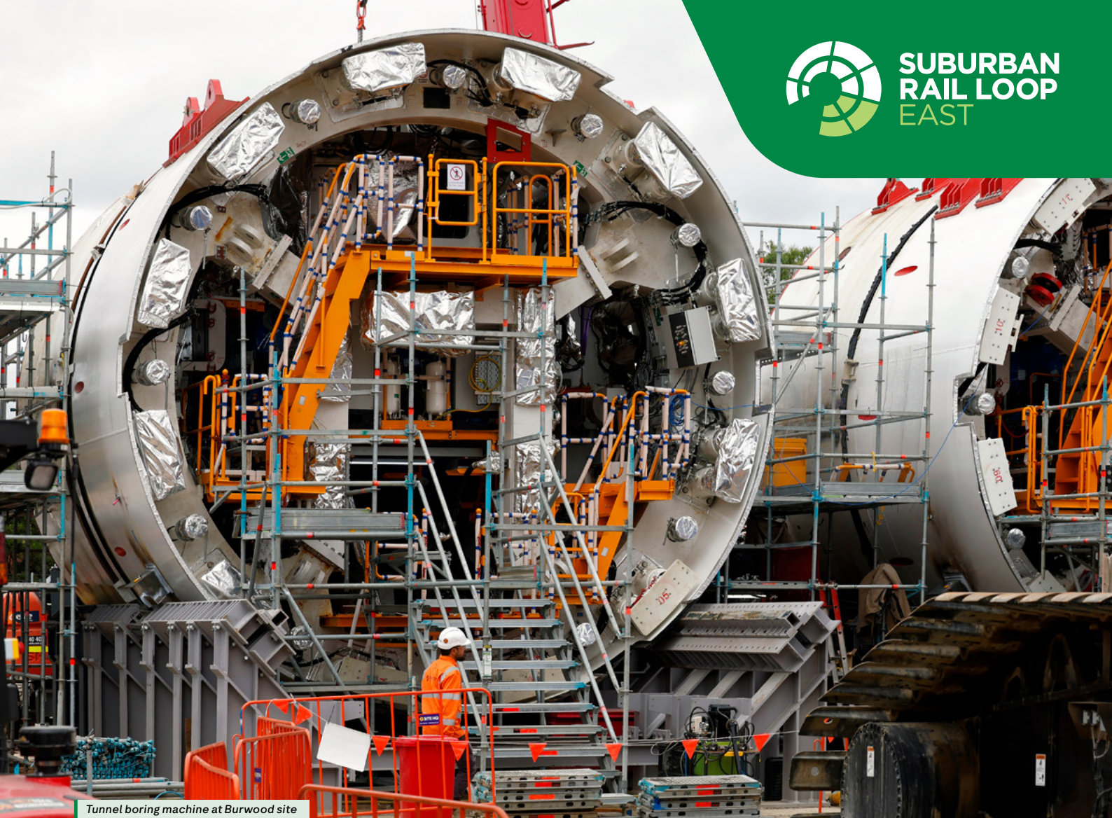
Tunnel boring machine at Burwood site
