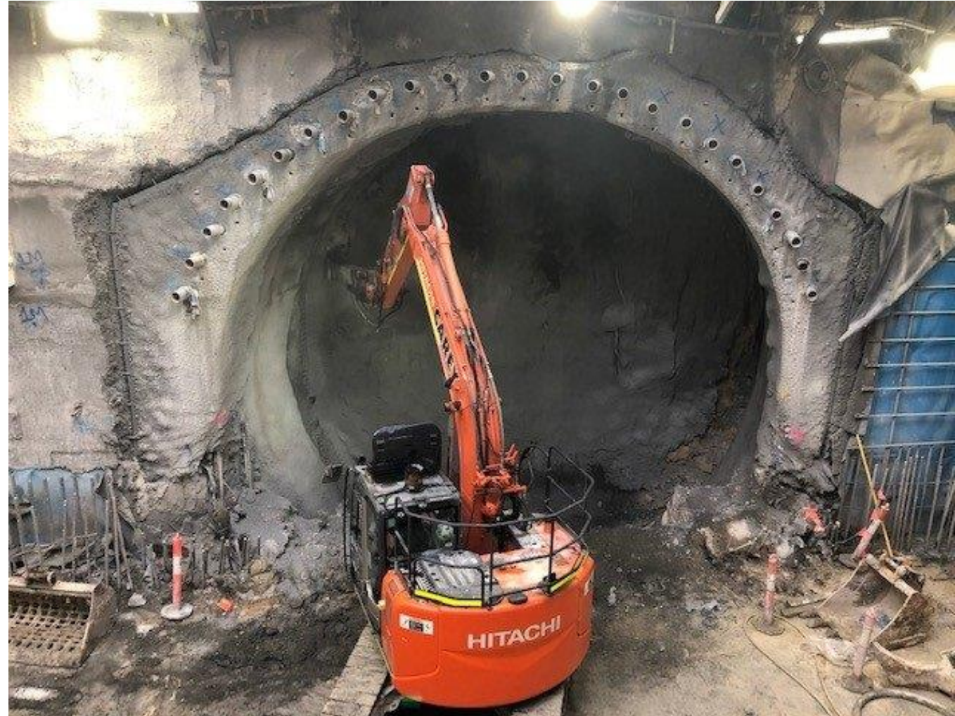
The eastbound stub tunnel in August
