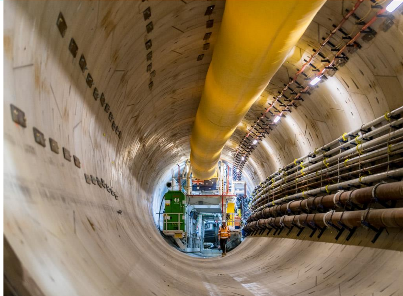
Alice & the westbound tunnel
