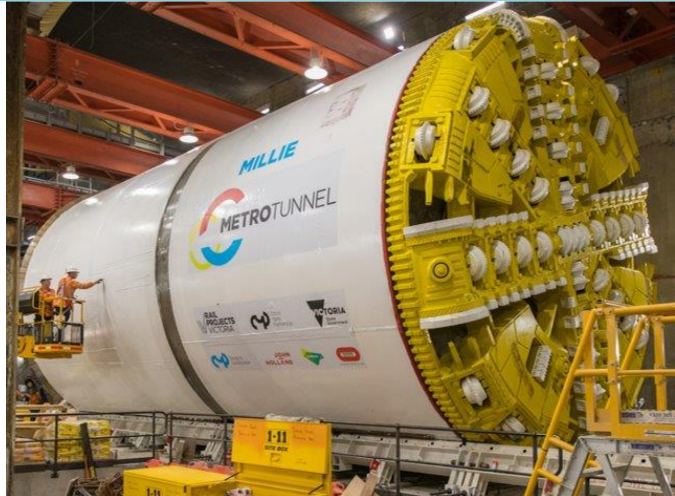
TBM Millie inside the Anzac Station box
