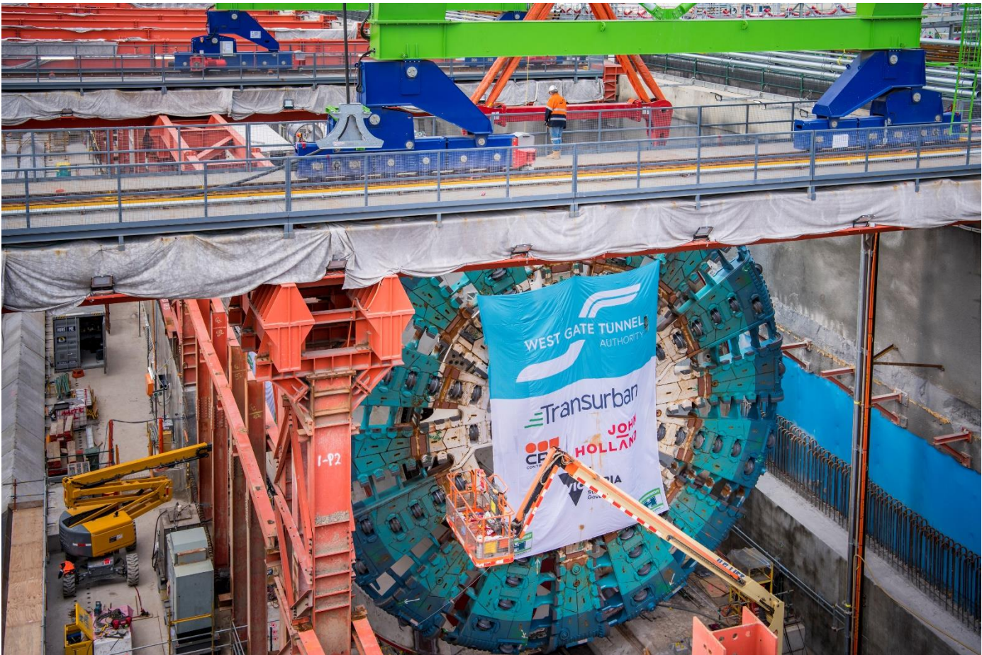
Photo 8 – Attachment of TBM cutter head to TBM body – Tunnel Zone (Source: WGTP MTIA, 29 August 2019)
