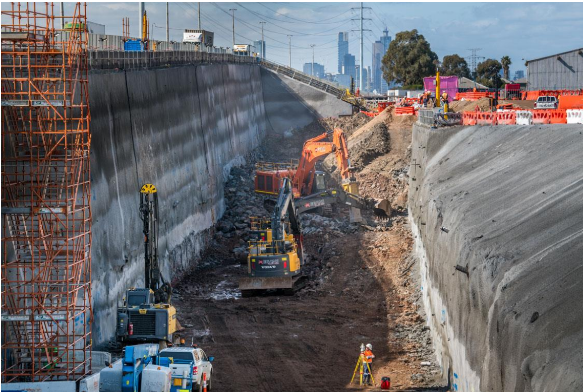
Photo 6 – South Portal bulk excavation – Tunnel Zone (Source: WGTP MTIA, 29 August 2019)
