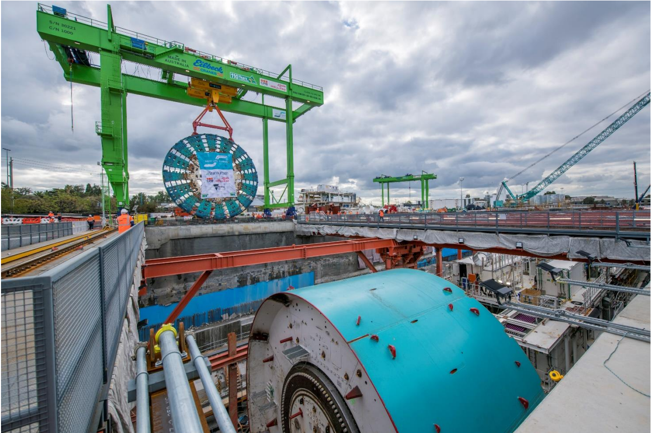
Photo 7 – Gantries lifting TBM cutter head – East Zone (Source: WGTP MTIA, 29 August 2019)
