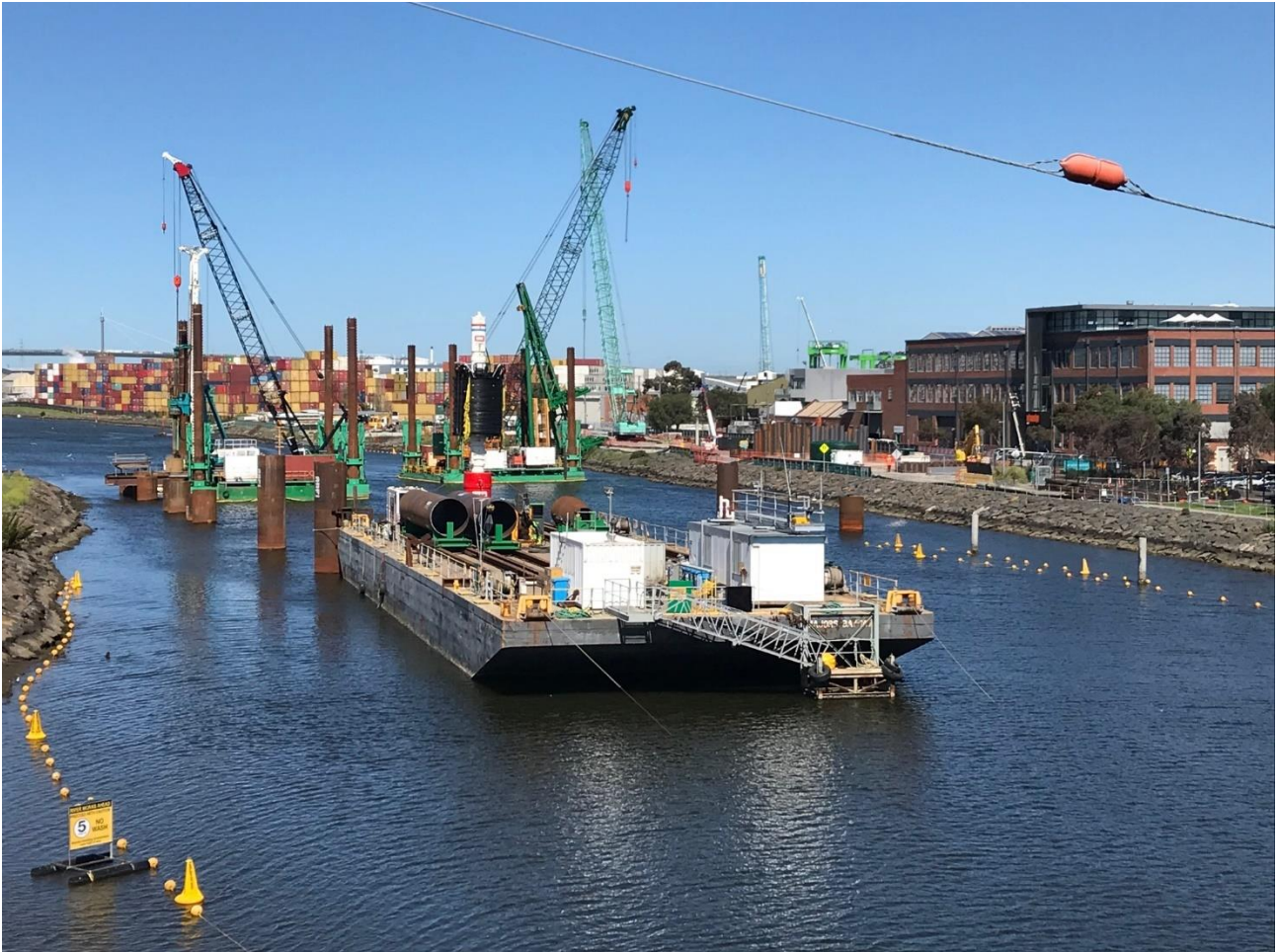
Photo 1 – Maribyrnong River pile driving – East Zone (Source: IREA, 20 September 2019)
