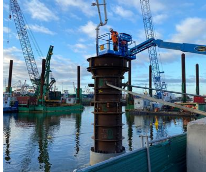
Concreting first marine column
