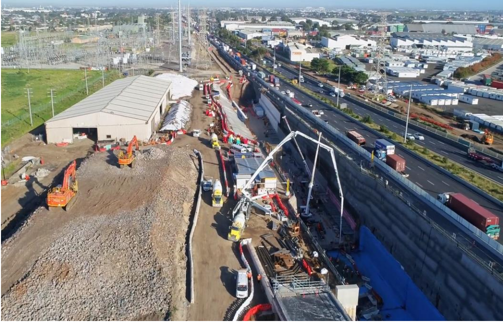
Excavation works at the Outbound South Portal
