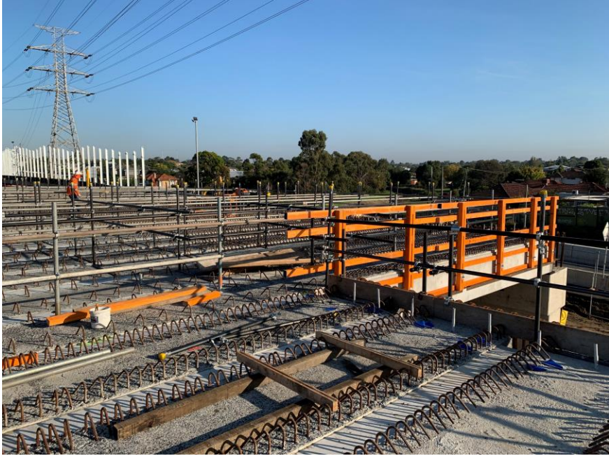
Pre-cast roof beams installed at the Inbound South Portal
