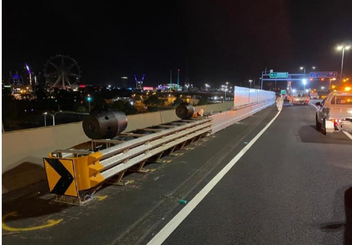
New barrier installation on CityLink at the Footscray Road off ramp.
