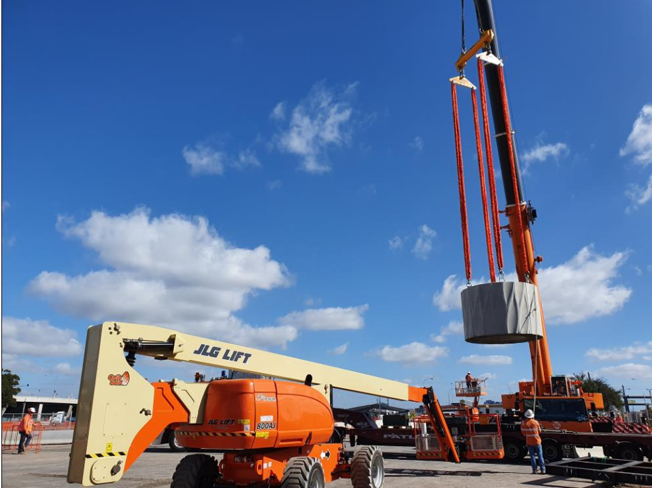
Pre-cast column segments being installed at the Fish Market site
