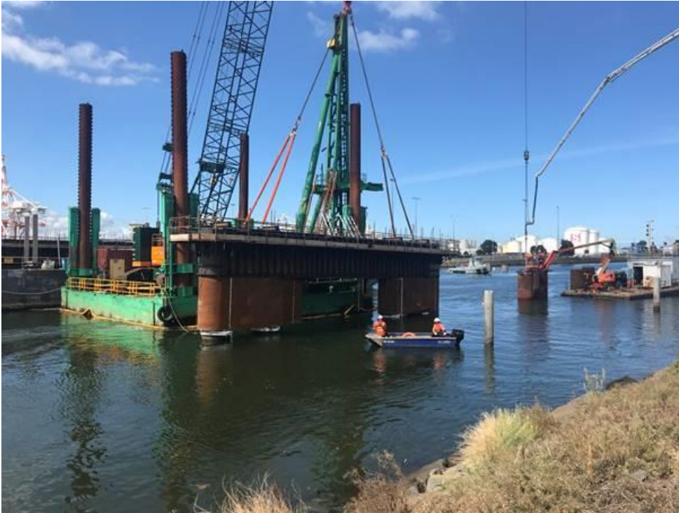
Installation of first marine tie beam formwork
