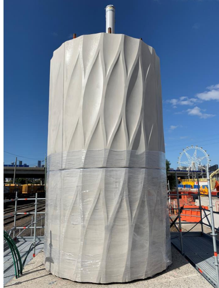
Pre-cast column segments being installed at the Fish Market site
