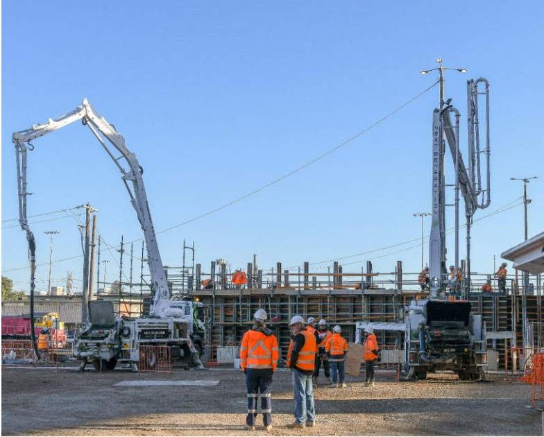
Pile cap being poured
