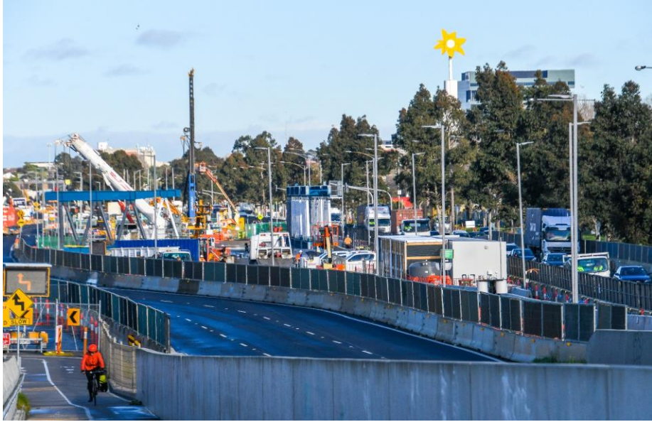
Footscray Road traffic switch and centre median construction site
