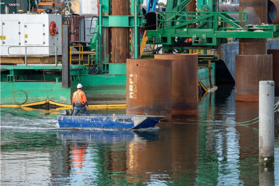
Inspecting the marine piles
