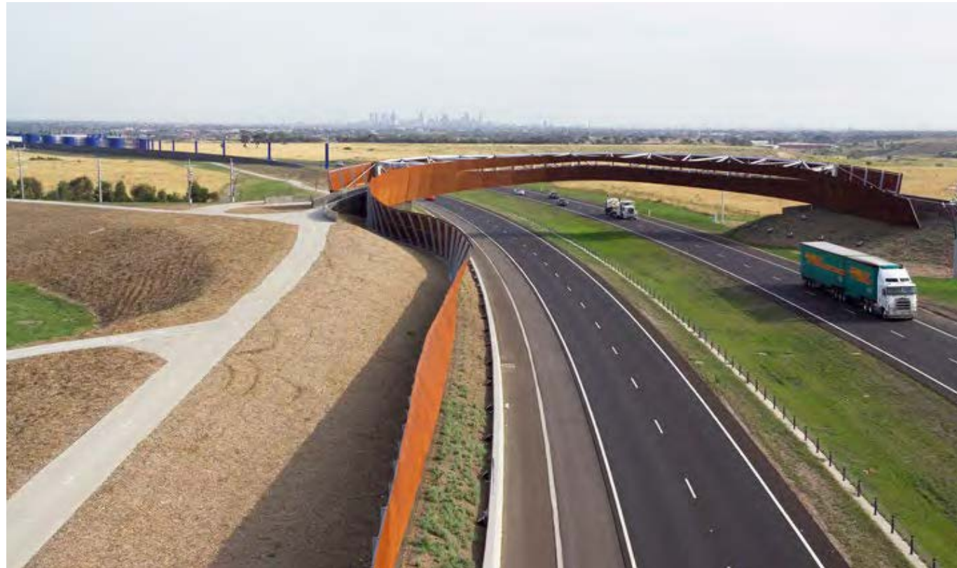
FIGURE 69 Demonstrates: integrated pedestrian bridge with noise walls to create a gateway that frames Melbourne's skyline. Craigieburn Bypass, Melbourne. Design: Taylor Cullity Lethlean, Tonkin Zulaikha Greer Architects and Robert Owen, Image: VicRoads
