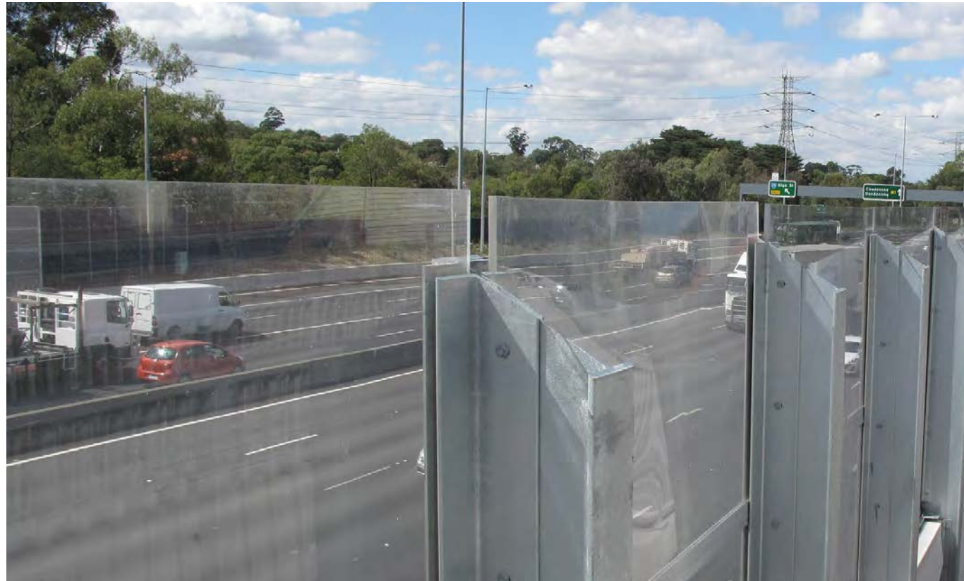
FIGURE 86 Demonstrates: transparent and clear noise walls minimise overshadowing and provide views to landscape outside the freeway reserve. M1 Monash York St Pedestrian bridge, Melbourne. Image: VicRoads
