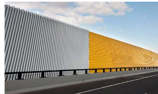
FIGURE 38 Demonstrates: transition of noise wall types (on and off structure noise walls with continuous protection barrier). Deer Park Bypass, Melbourne. Design: Peter Elliott, Image: VicRoads, Photography: John Gollings
