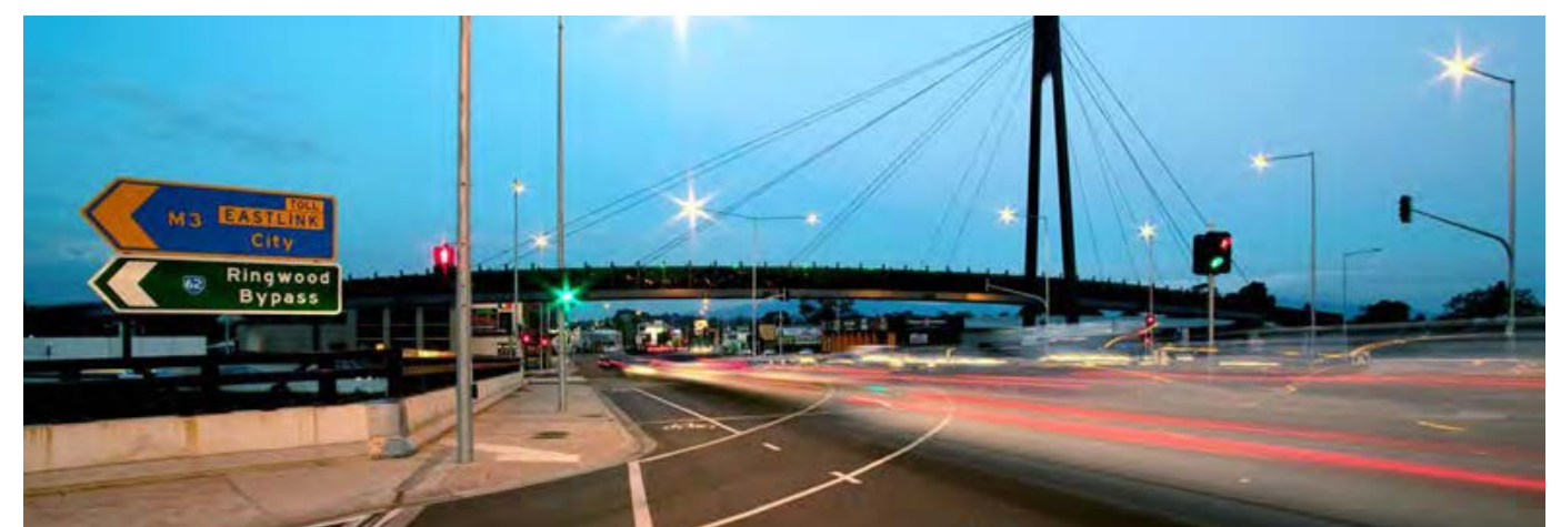
FIGURE 65 Demonstrates: cable stay pedestrian bridge that creates a landmark for travellers and eliminates the requirement for roadside barriers. EastLink, Melbourne. Design: Wood Marsh, Image: GHD
