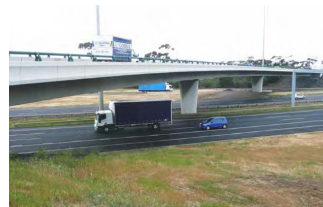
FIGURE 5 Demonstrates: a continuous and streamlined pier and box girder bridge structure design. Image: VicRoads
