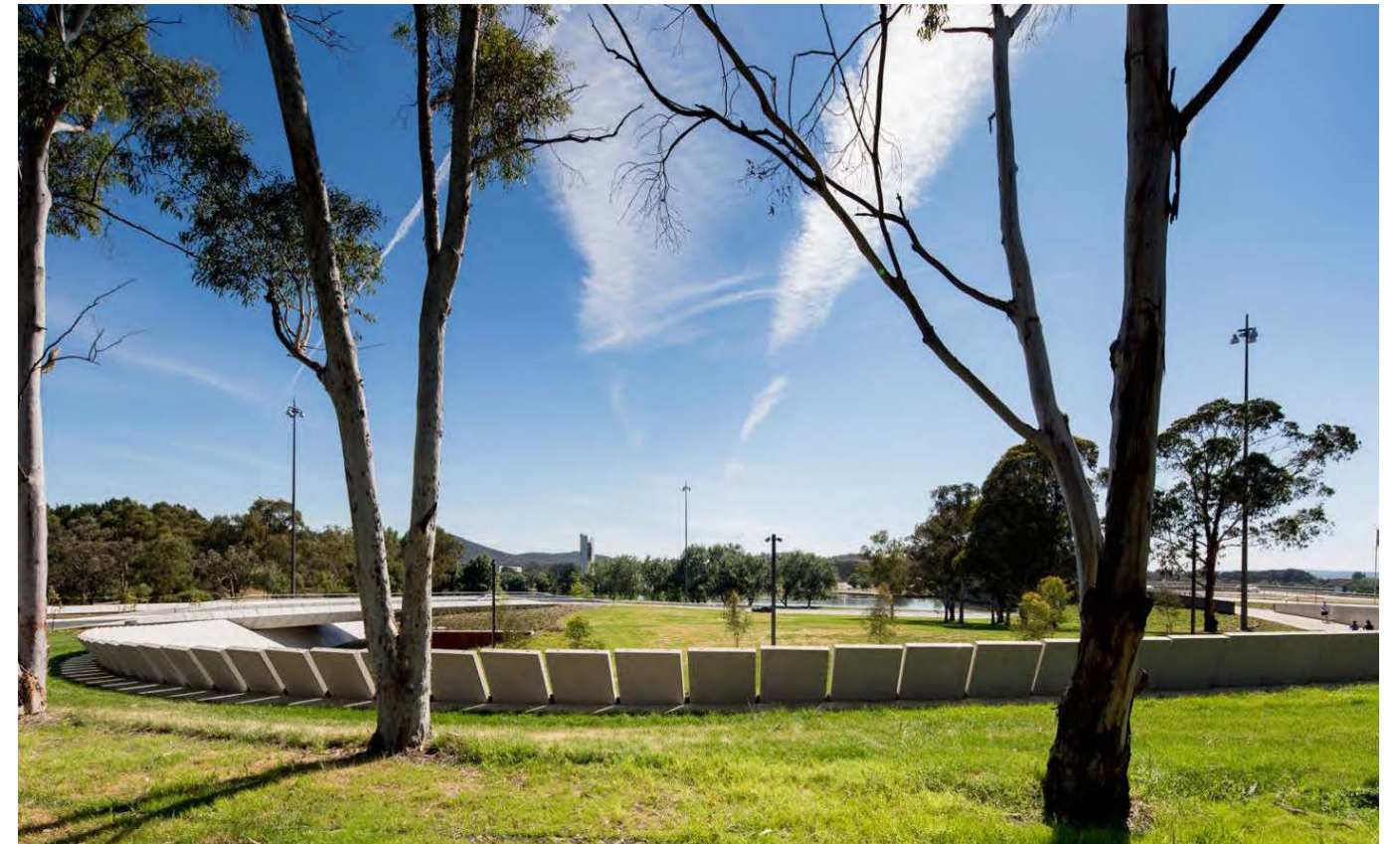
FIGURE 67 Demonstrates: well integrated retaining walls extended to address safety as part of the design. Design: Lahz Nimmo Pty Ltd and Spackman Mossop Michaels, Photography: Brett Boardman
