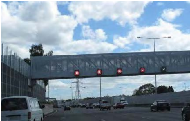
FIGURE 84 Demonstrates: LUMS (land use management) integrated with pedestrian bridge. M1 York Street pedestrian bridge, Melbourne. Design: Denton Corker Marshall, Image: VicRoads
