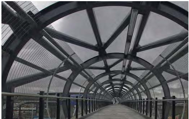
FIGURE 59 Demonstrates: integration of screens into the form of the pedestrian bridge. Williams Landing Train Station, Melbourne. Design: Arup and Cox, Image: VicRoads
