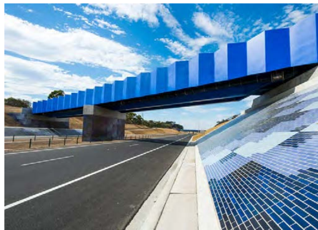
FIGURE 7 Demonstrates: a solution to abutment design that assists in creating a family of bridges. Peninsula Link Melbourne. Design: ARM Architecture, Image: Southern Way
