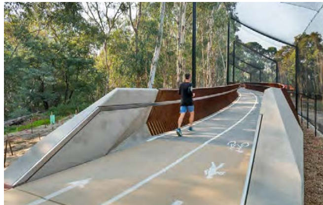
FIGURE 61 Demonstrates: well integrated interface between pedestrian bridge and adjoining path. Darebin Yarra Trail, Melbourne. Design: VicRoads, Photography: Emma Cross
