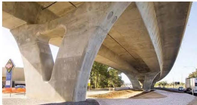
FIGURE 1 Demonstrates: well considered pier forms integrated with super structure, providing clear visual permeability across the ground plane. South Road Superway, Adelaide. Image: GHD
