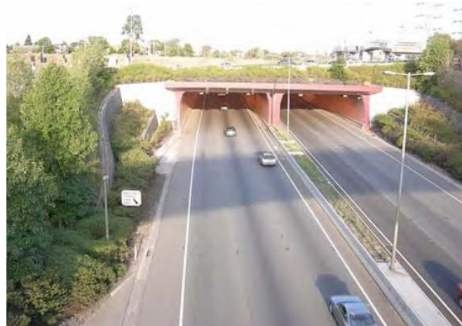
FIGURE 73 Demonstrates: use of vegetation to soften tunnel entry. M80 Jacana Tunnel entry in Pascoe Vale, Melbourne. Image: VicRoads
