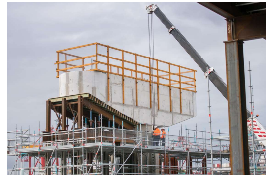
Concrete and steel installation on Footscray Road to support the future elevated roadway
