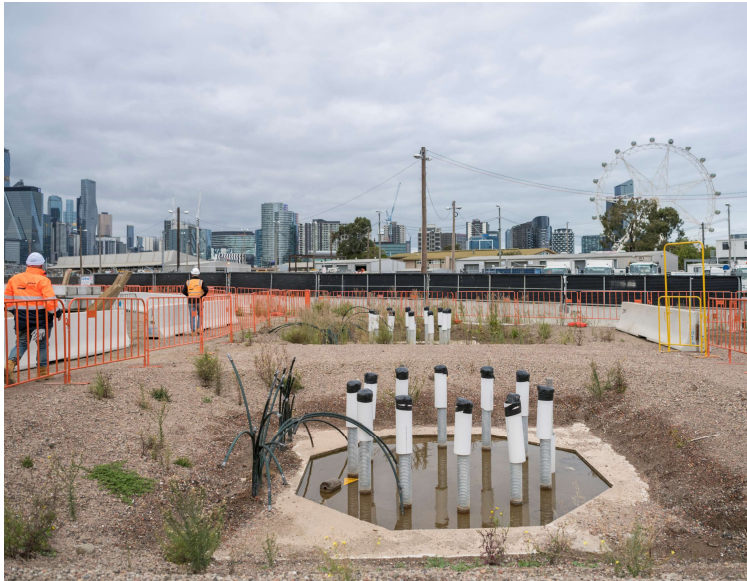
Pile caps completed for the Southbound carriageway
