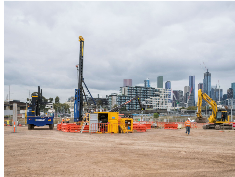
Driven piling being completed for the North and Southbound carriageway
