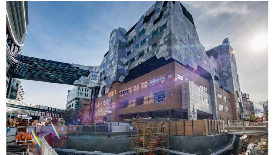
Grattan Street West Works
