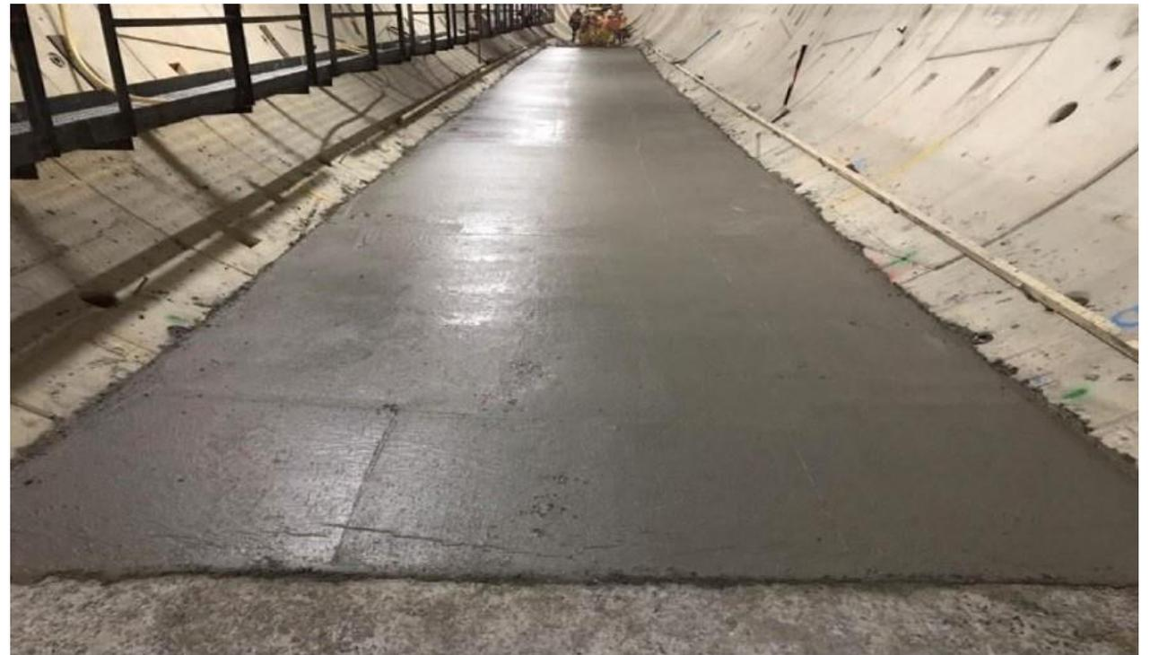
*A section of first stage concrete invert works in eastbound tunnel*
