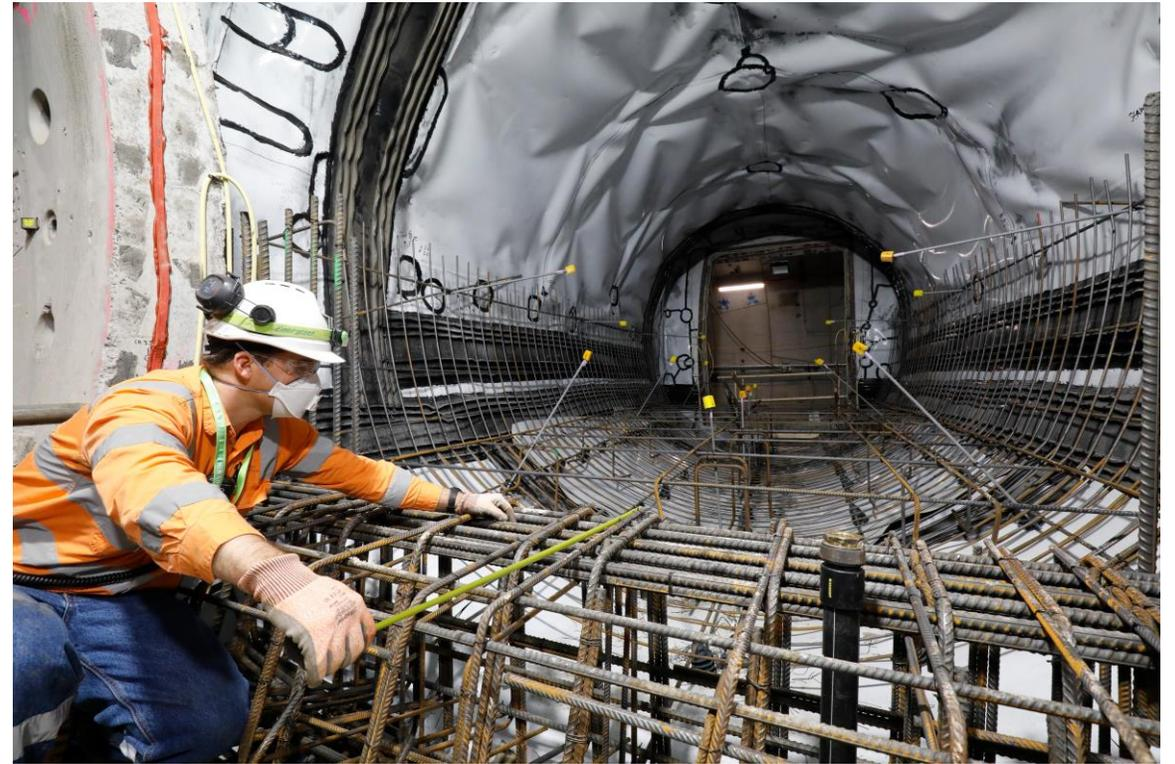
*Waterproofing and lining works at one of the remaining cross passages*
