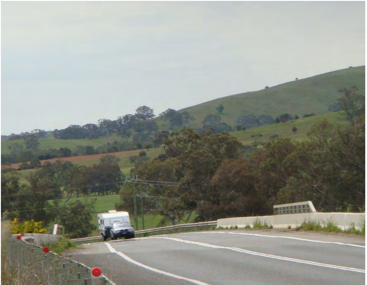
Western Highway, Armstrong Deviation - looking north
