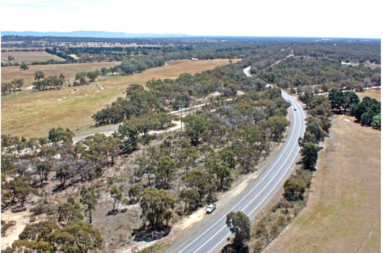
Western Highway, Oddfellows Bridge - looking north
