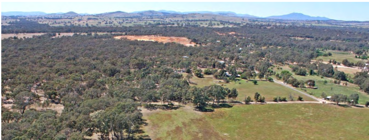
Existing Quarry, north-east of Great Western
