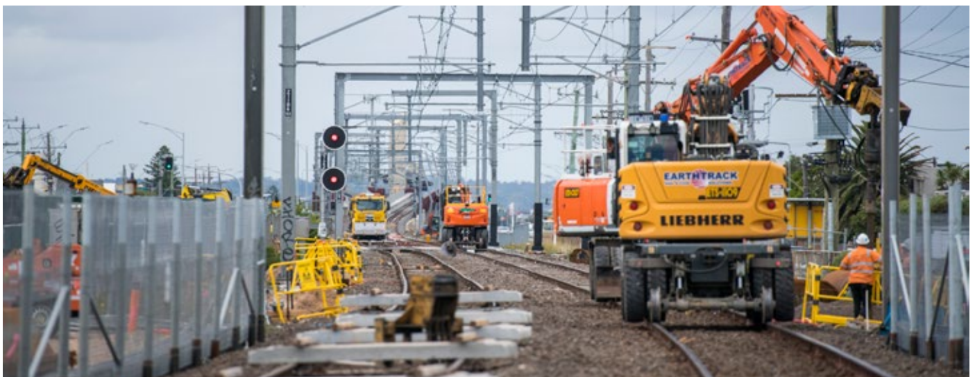
Crews replacing rail sleepers along the rail line between Edithvale and Bonbeach during our February rail closure
