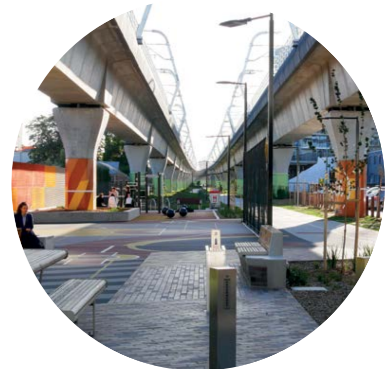
New community space underneath an elevated rail bridge in Carnegie
