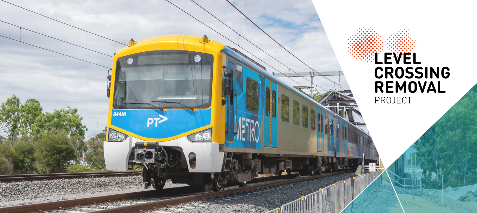
Train running over the new, duplicated tracks at Eumemmerring Creek bridge
