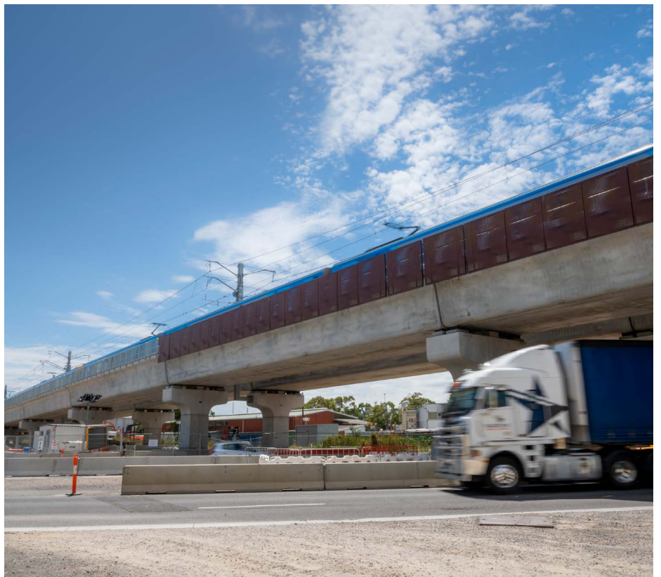
Cars travelling underneath the new Greens Road rail bridges
