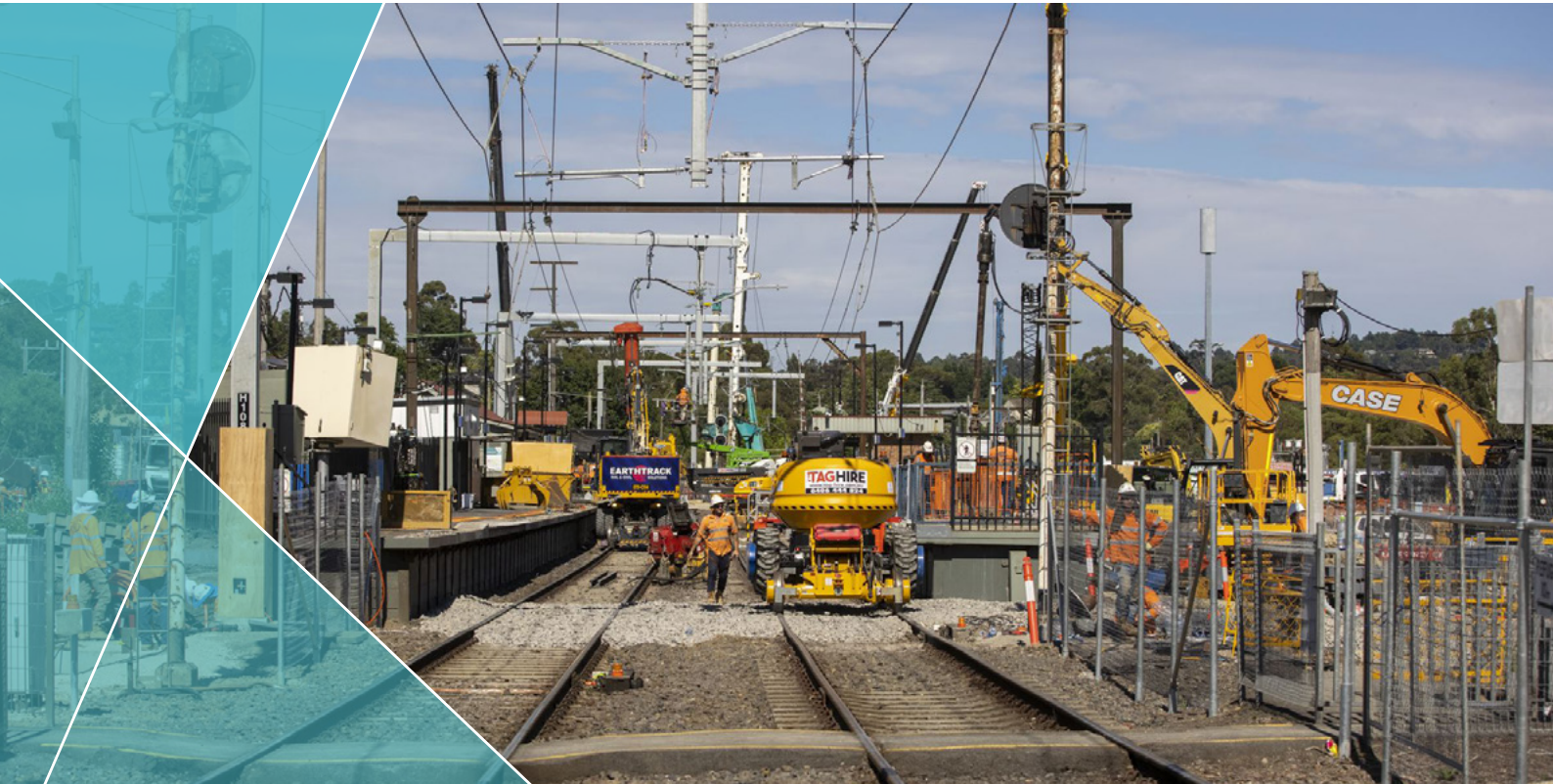
Construction to remove the Manchester Road, Mooroolbark level crossing
