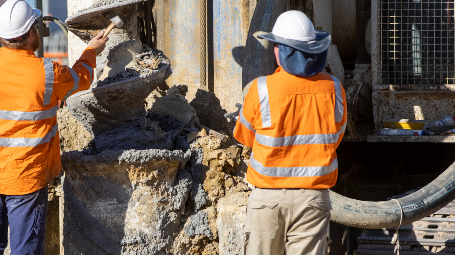
Piling rig used to dig foundations at Manchester Road, Mooroolbark
