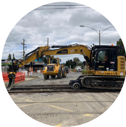
Heavy machinery to remove track at Manchester Road, Mooroolbark
