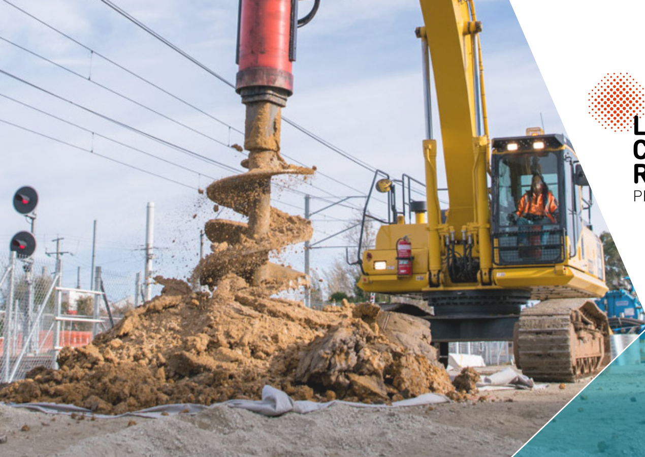
Piling rig drilling into the earth.
