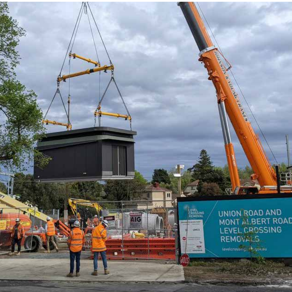
Prefabricated station building being lifted into place for the new Union Station
