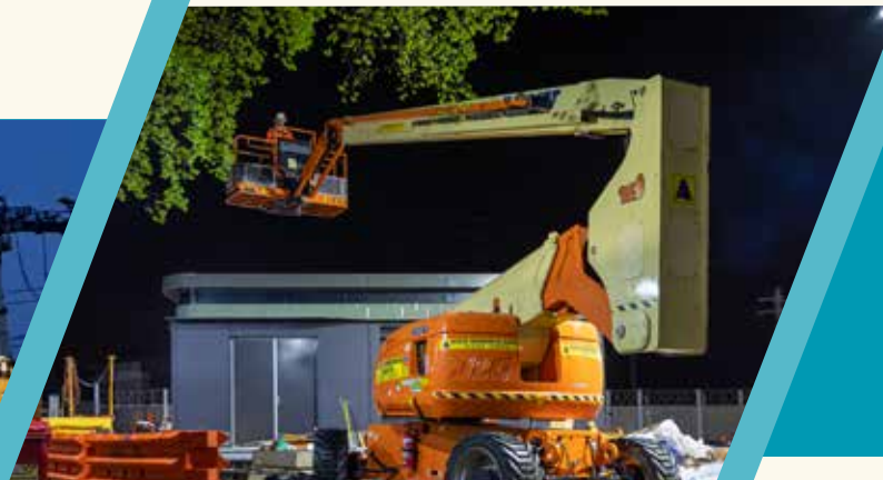
Station building in place
