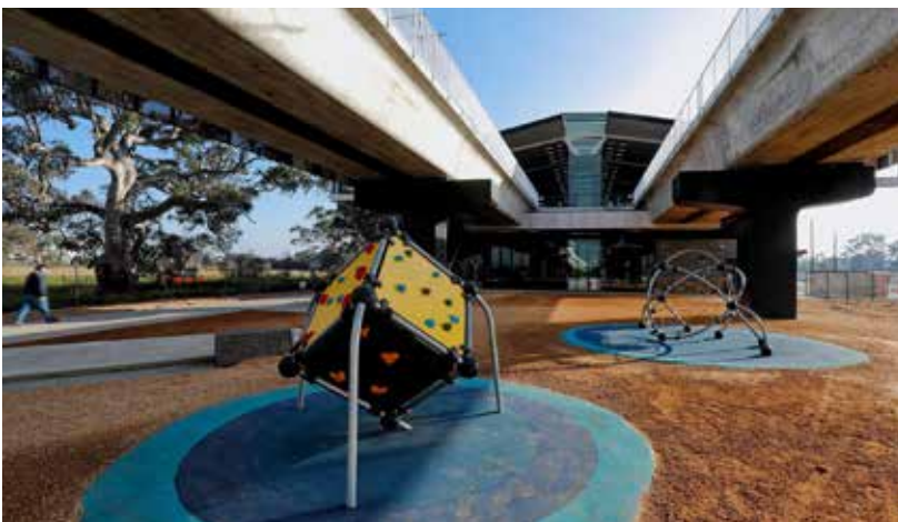
Community space at Mernda Station
