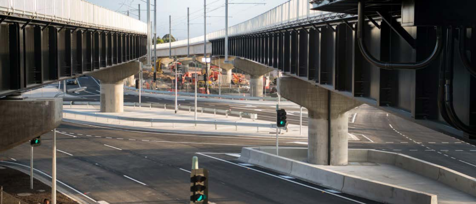
Example of steel bridge at High Street, Reservoir.
